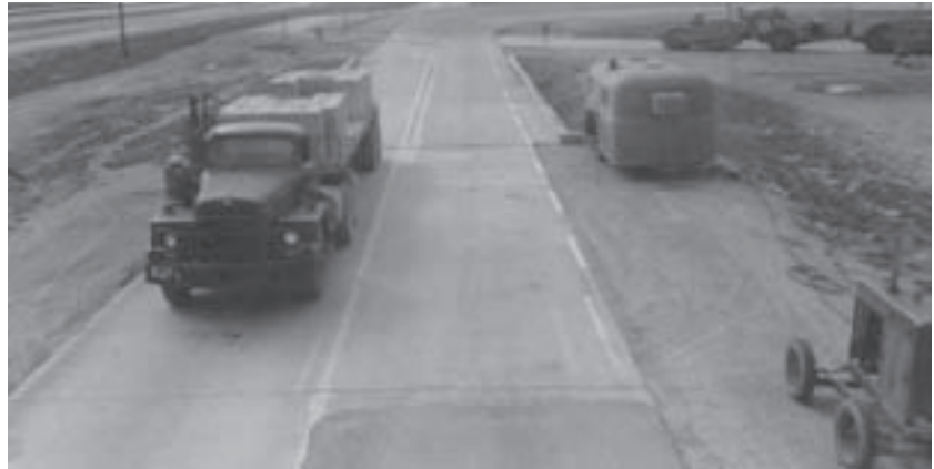
Loaded truck crosses test bridge. Bridge trailer that housed data recorders is at right.
