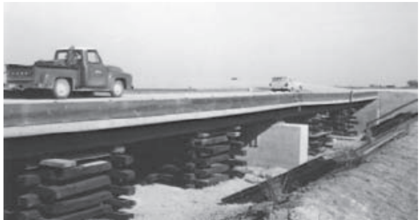
Cribbing placed below test bridges.
