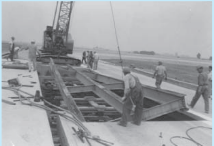
Removing damaged steel from test bridge.
