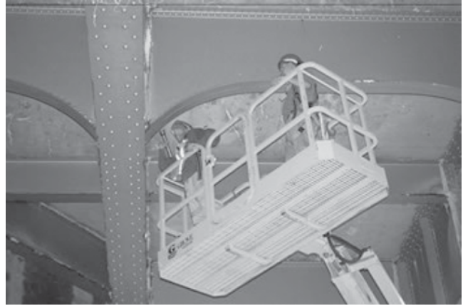
FIGURE 6 Hands-on inspection from manlift.
