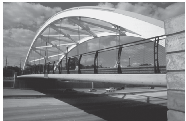
FIGURE A13 Post-tension tied arch bridge in Houston, Texas.
