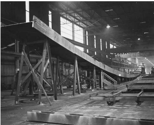
FIGURE 6 Progressive girder assembly.
