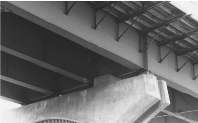
FIGURE 2 Deck cantilever brackets (DeLong's Inc.).
