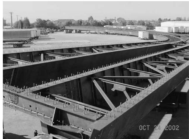
FIGURE 7 Special complete structure assembly (Washington State DOT).
