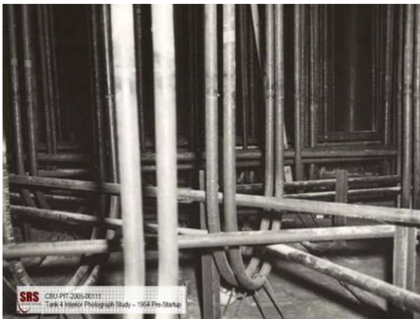
FIGURE 4 Photograph of the interior of a Type I tank (Tank 4) prior to receipt of wastes. SOURCE: Caldwell (2005a).
