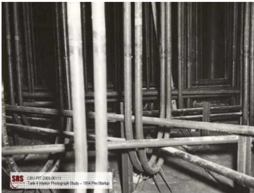
FIGURE S-1 Photograph of the interior of a Type I tank (Tank 4) prior to receipt of wastes.
