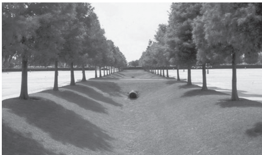
FIGURE 3.5 Rain gardens and street medians used for water drainage not only store water but provide rich and beautiful ecological zones. SOURCE: Tom Fox, the SWA Group. Reprinted with permission.
