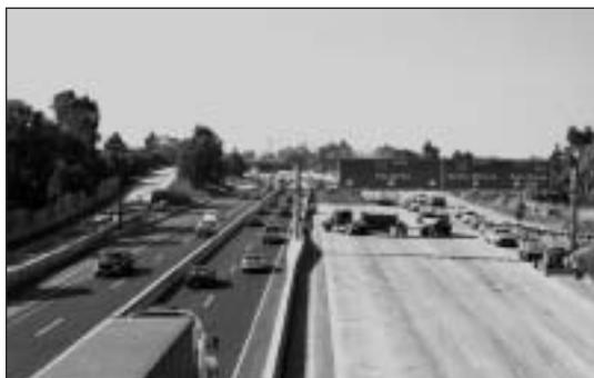
A longlife asphalt concrete project on the Long Beach Freeway in California exemplifies the “get in, get out, stay out” approach for highway construction.
