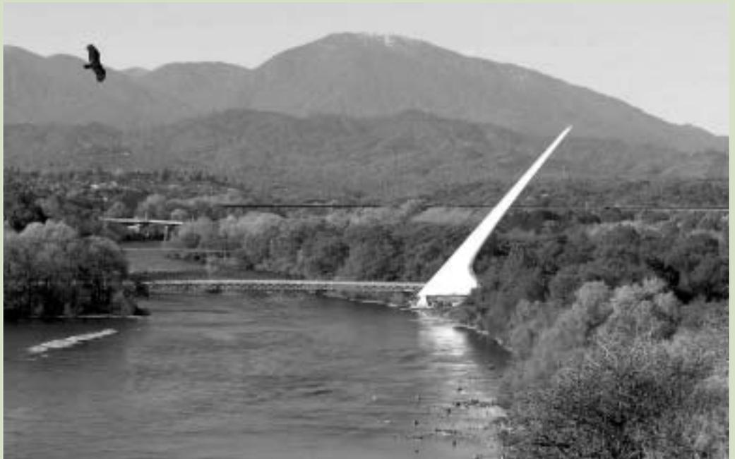
and transported by truck to Redding. The parts, supported by cables stretched from the pylon, were welded together above the water.
