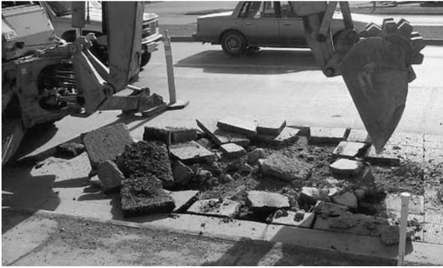
FIGURE 39 UTW repair step 2—Removing panels.
