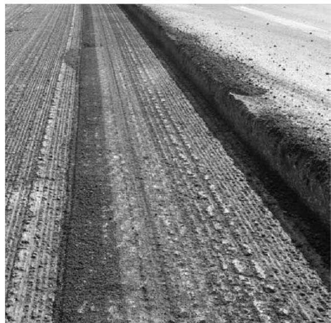
FIGURE 7 Milled HMA surface before overlay.
