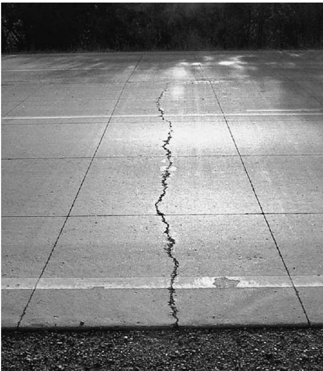
FIGURE 32 Typical midpanel crack on a TWT.
