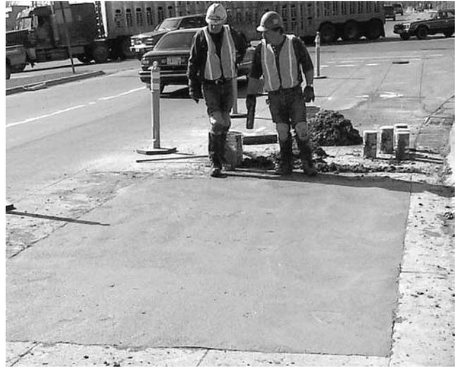
FIGURE 41 UTW repair step 4—Finish and cure PCC.
