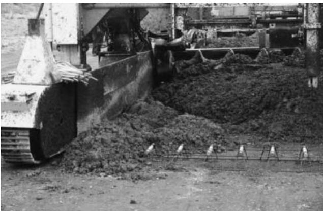
FIGURE 15 Concrete being placed over a dowel basket.
