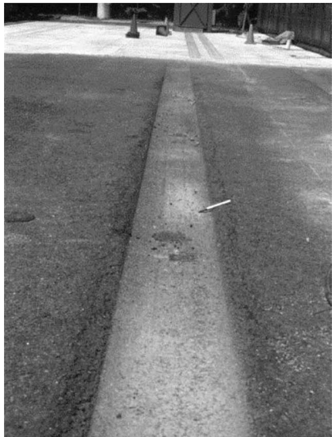
FIGURE B16 Typical HMA rutting at the FHWA ALF.
