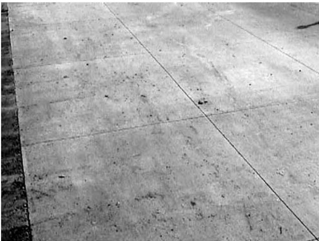
FIGURE 26 Joints without joint sealant.
