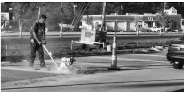
FIGURE 24 Sawcutting on a fast-tracked UTW.
