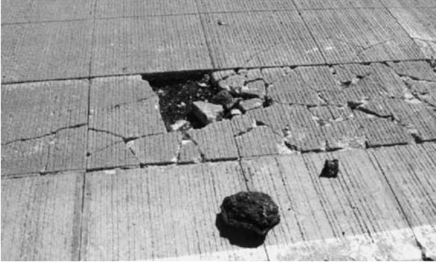
FIGURE 35 Severely shattered slabs on a UTW.
