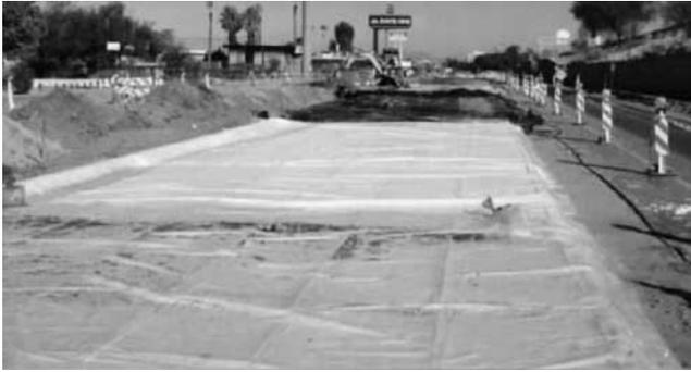
FIGURE 23 Polyethylene sheeting used as a curing method.
