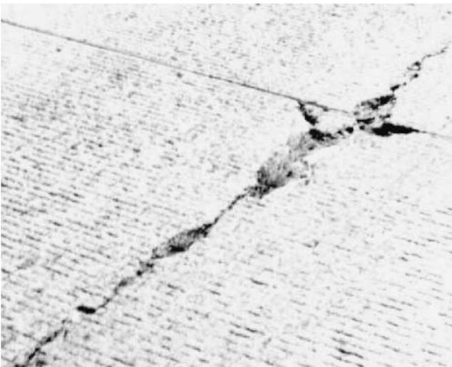
FIGURE 36 Severely spalled crack.
