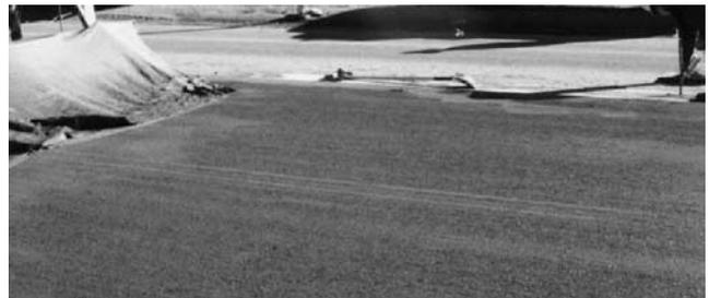
FIGURE 19 Application of texture with a burlap drag.
