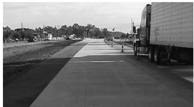
FIGURE 27 New shoulders meeting a new whitetopping elevation.
