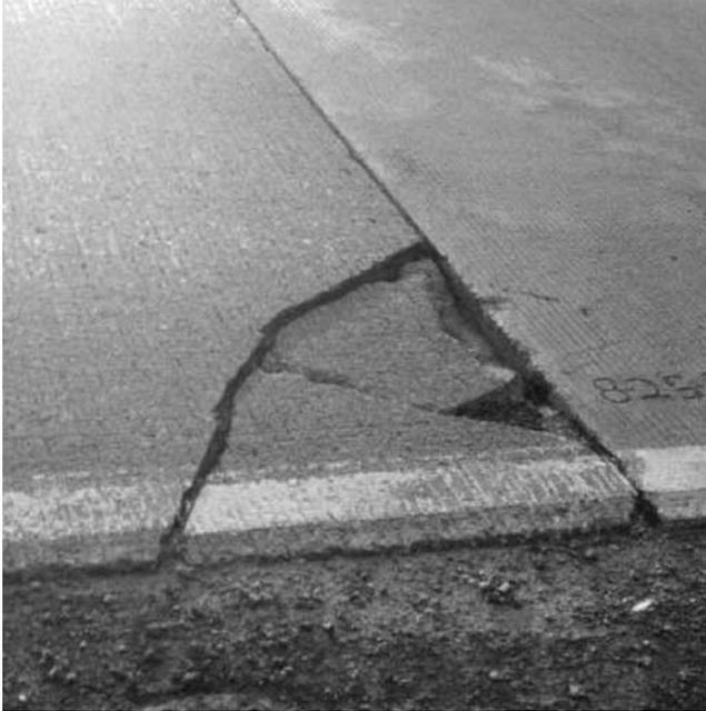
FIGURE 31 Deteriorated corner crack on a TWT.
