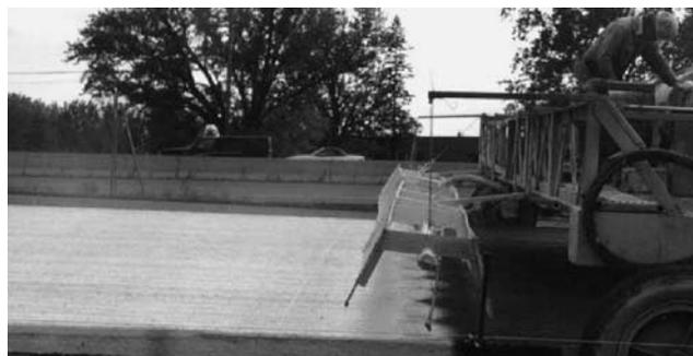
FIGURE 22 White-pigmented, liquid membrane curing compound.
