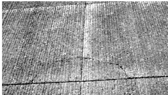
FIGURE 30 Typical corner crack on a UTW.
