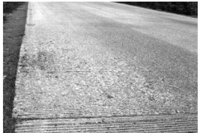
FIGURE 37 Typical surface wear.
