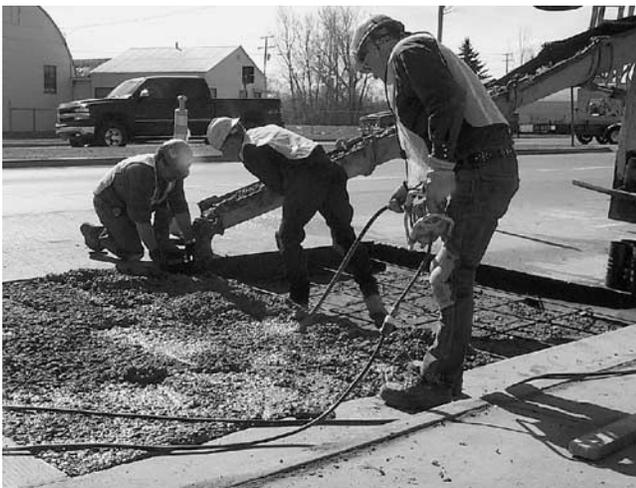
FIGURE 40 UTW repair step 3—Place new PCC.
