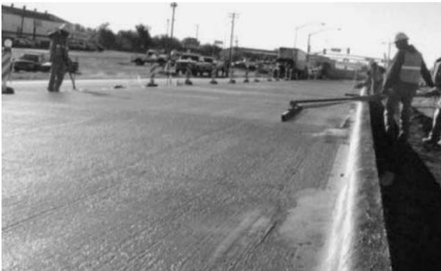
FIGURE 18 Water sheen on a concrete surface.
