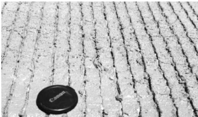
FIGURE 21 Tining comb texturization on freshly placed concrete.
