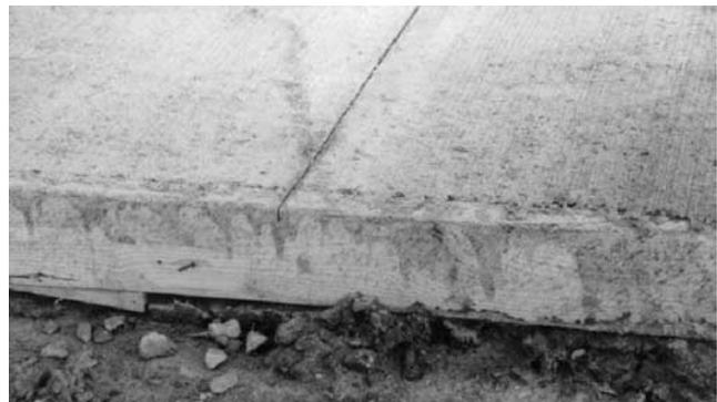
FIGURE 25 Sawcut depth using an early-age saw.
