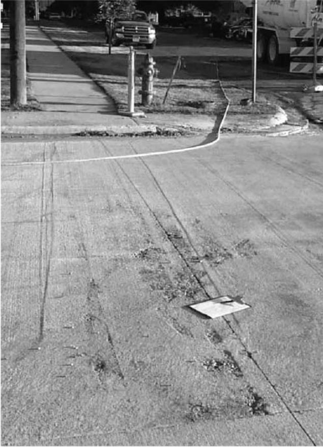
FIGURE 14 Poor consolidation.
