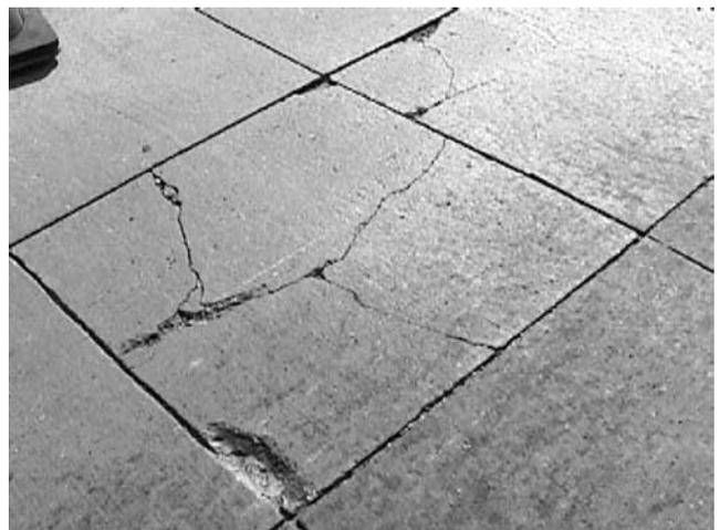
FIGURE 34 Typical shattered slab on a UTW.
