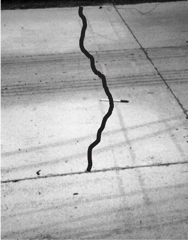
FIGURE B12 Typical UTW transverse cracking at the FHWA ALF.
