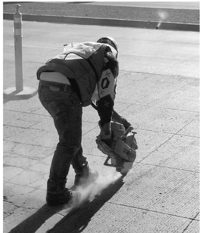
FIGURE 38 UTW repair step 1—Outline sawing.
