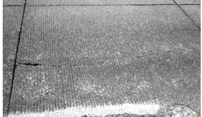
FIGURE 33 Typical midpanel crack on a UTW.
