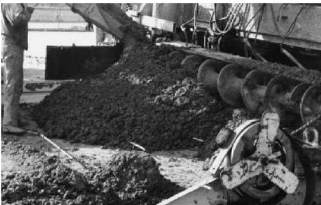
FIGURE 12 Use of a slipform paver.
