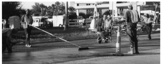
FIGURE 20 Application of texture with a coarse broom.
