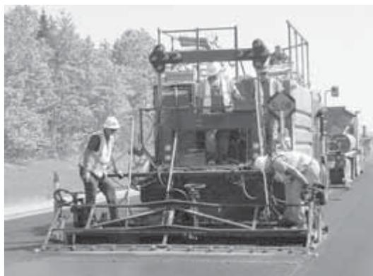
Microsurfacing is one of many pavement preservation techniques that states are integrating into a plan of preventive maintenance, rehabilitation, and reconstruction.
