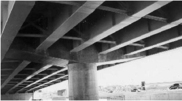
*Figure 1. Concrete pier cap connected integrally to steel I-girder superstructure.*
