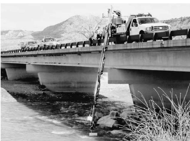
Figure B2. Using the articulated arm to sweep arc's on the upstream side of bridge.
