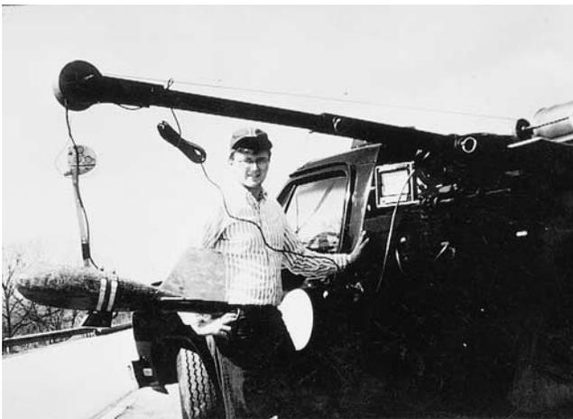
Figure 1. USGS type stream gaging crane being used for scour monitoring.
