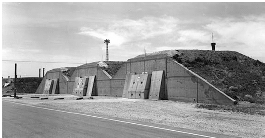
FIGURE 2-3 Storage bunkers at the Pantex weapon assembly plant in Texas.
