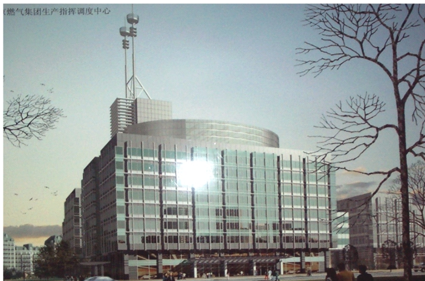
FIGURE 1 The Beijing Gas Group Office Building (23,000 m 2 ) is already built and is being commissioned. Major energy equipment includes: 1 set of 480 kW + 1 set of 72 kW Caterpillar gas engines; and 1 set of BZ100 + 1 set of BZ200 waste-heat direct-absorption gas turbines. The system guarantees basic power needs. Any shortfall for heating, cooling, or hot water is supplied by the grid.
