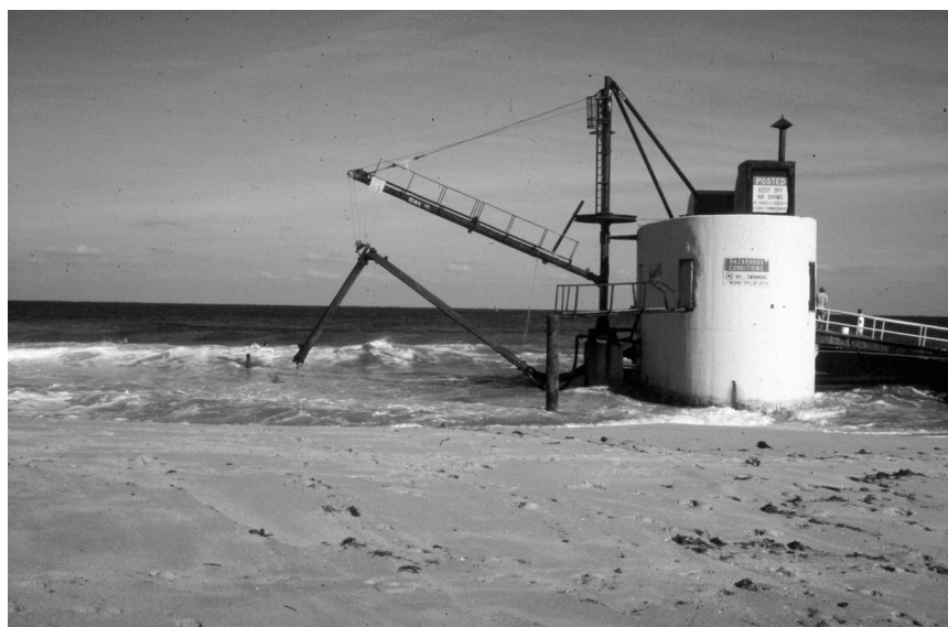
FIGURE 2-6 Port of Palm Beach, Lake Worth Entrance sand transfer plant. Photo courtesy of Robert Dean, University of Florida.
