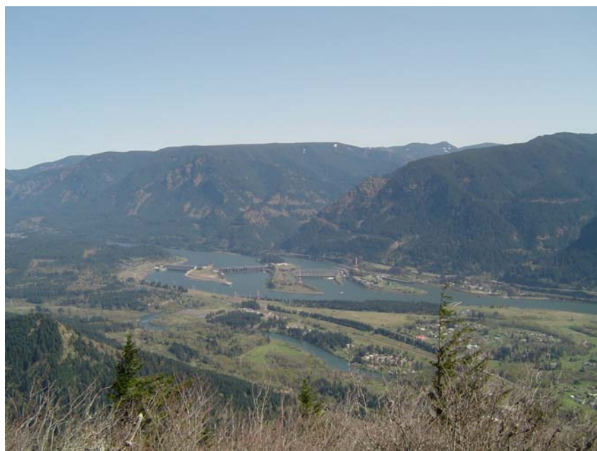
View of Bonneville Dam, with its spillway and two powerhouses. Photo courtesy of Jeffrey Jacobs.
