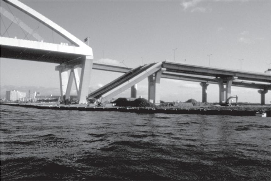
FIGURE 2.8 Failure of a span of the Nishinomiya Bridge during the 1995 Kobe, Japan, earthquake. Reproduced courtesy of the National Information Service for Earthquake Engineering, University of California, Berkeley.
