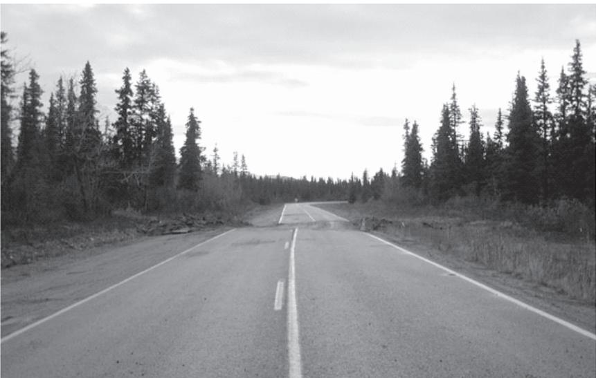
FIGURE 2.9 Lateral highway offset of 2.5 meters as a result of the 2002 Denali, Alaska, Earthquake. SOURCE: Alaska Department of Natural Resources. Photo by Patty Craw, Division of Geological and Geophysical Surveys.
