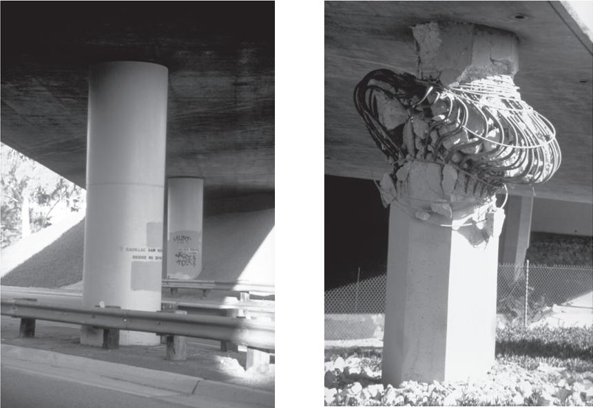
FIGURE 1.2 Comparison of retrofitted and unimproved concrete bridge columns following the 1994 Northridge, California, earthquake. *Left:* Cadillac Avenue ramp at Interstate 10 (Santa Monica Freeway). *Right:* Highway 118/Bull Creek Bridge. Reproduced courtesy of the National Information Service for Earthquake Engineering, University of California, Berkeley.
