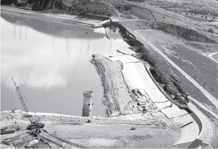
FIGURE 2.4 Embankment failure due to liquefaction at the Lower Van Norman Dam, 1971 San Fernando, California, earthquake. Reproduced courtesy of the National Information Service for Earthquake Engineering, University of California, Berkeley.
