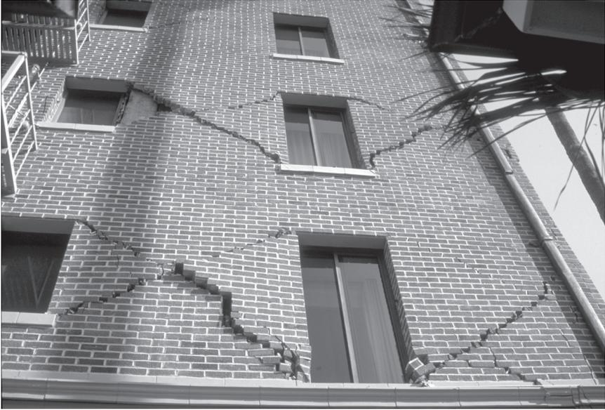
FIGURE 2.6 Structural damage to masonry building resulting from the 1994 Northridge, California, earthquake. Reproduced courtesy of the National Information Service for Earthquake Engineering, University of California, Berkeley.
