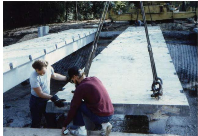
FIGURE 33 Construction of transversely posttensioned double-tees bridges.
