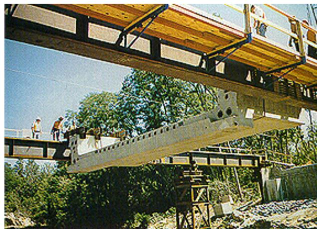
FIGURE 4 Installation of the first two channel segments of the Carpenter Road Bridge. (Source: <http://www.tfhrcc.gov/pubrds/septoct98/channel.htm>.)
