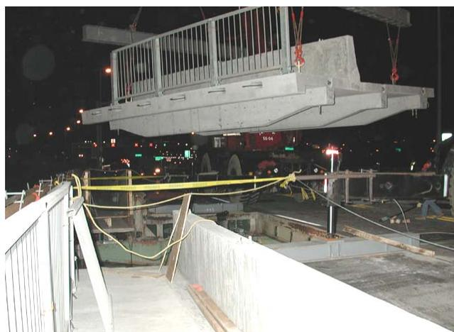
FIGURE 43 Prefabricated deck panel. (Source: [www.pjcci.ca](http://www.pjcci.ca).)
