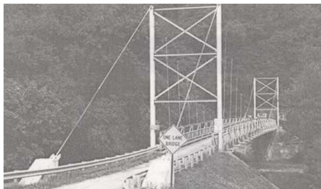
FIGURE 3 Corbin Bridge aluminum deck. (Source: [www.aluminum.org/Content/NavigationMenu/The\\_Industry/Building\\_Construction\\_Market/Bridges/Bridges.htm](http://www.aluminum.org/Content/NavigationMenu/The_Industry/Building_Construction_Market/Bridges/Bridges.htm).)
