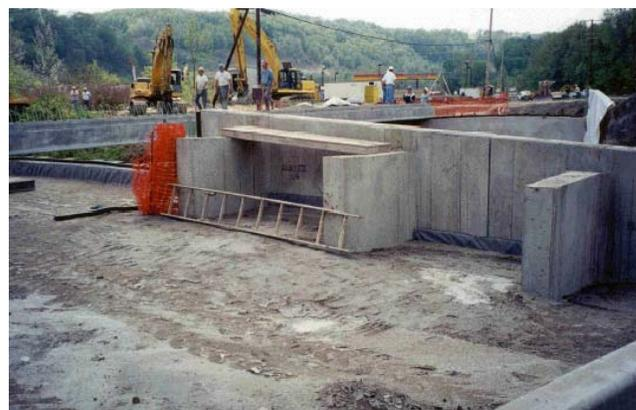
FIGURE 36 Fluid backfill behind abutment. [Source: Scanlon et al. (26).]
