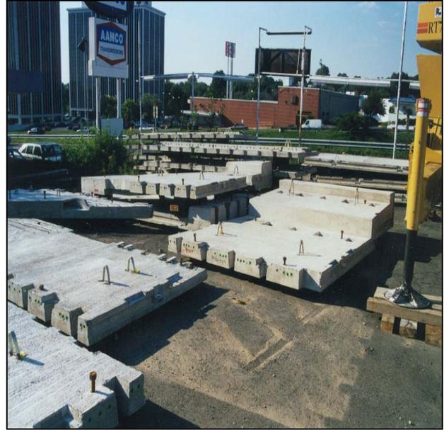
FIGURE 28 Stored panels near job site of bridges at Route 7 over Route 50, Fairfax, Virginia. [Source: Babaei et al. (1).]
