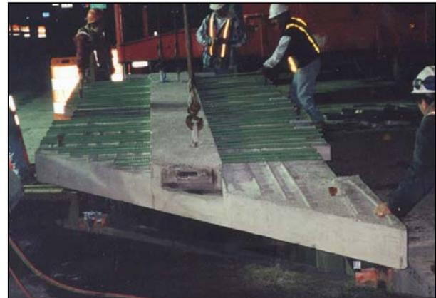
FIGURE 29 Installation of new panel of bridges at Route 7 over Route 50, Fairfax, Virginia. [Source: Babaei et al. (1).]
