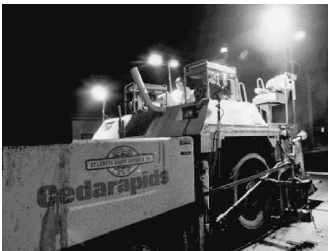
Figure 2. Typical paver operating with contractor-installed lighting (Buffalo, New York).
