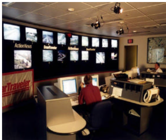
Figure 1: Intelligent Transportation System control facility. Source: Presentation by J. R. Thomas, June 13, 2003.
