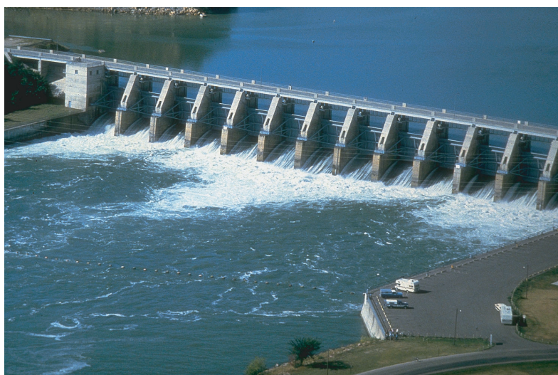
PHOTO 2.6 Gavins Point Dam (from Corps of Engineers Digital Visual Library http://images.usace.army.mil/ )
