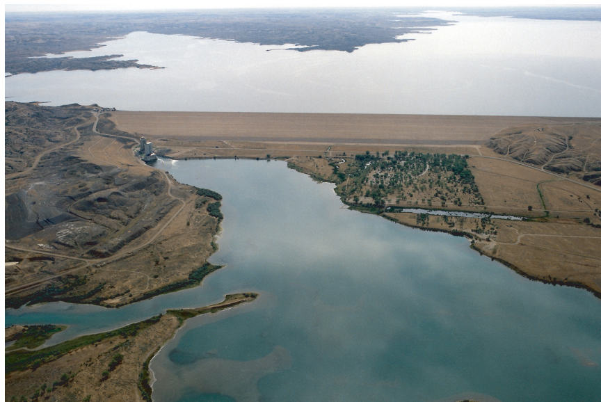
PHOTO 2.1 Fort Peck Dam (from Corps of Engineers Digital Visual Library http://images.usace.army.mil/ )
