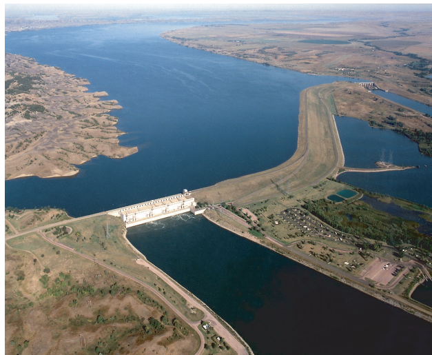
PHOTO 2.4 Big Bend Dam (from Corps of Engineers Digital Visual Library http://images.usace.army.mil/ )
