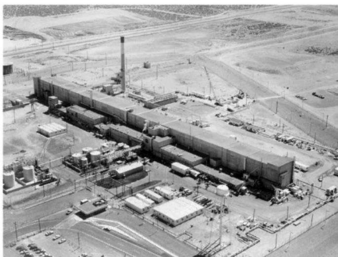
*FIGURE 2.4 Chemical separation of plutonium from other radioactive materials was carried out in Hanford's PUREX plant and similar facilities. They were referred to as canyons because thick walls to protect workers from radiation surrounded the long, remotely operated processing corridor.*
