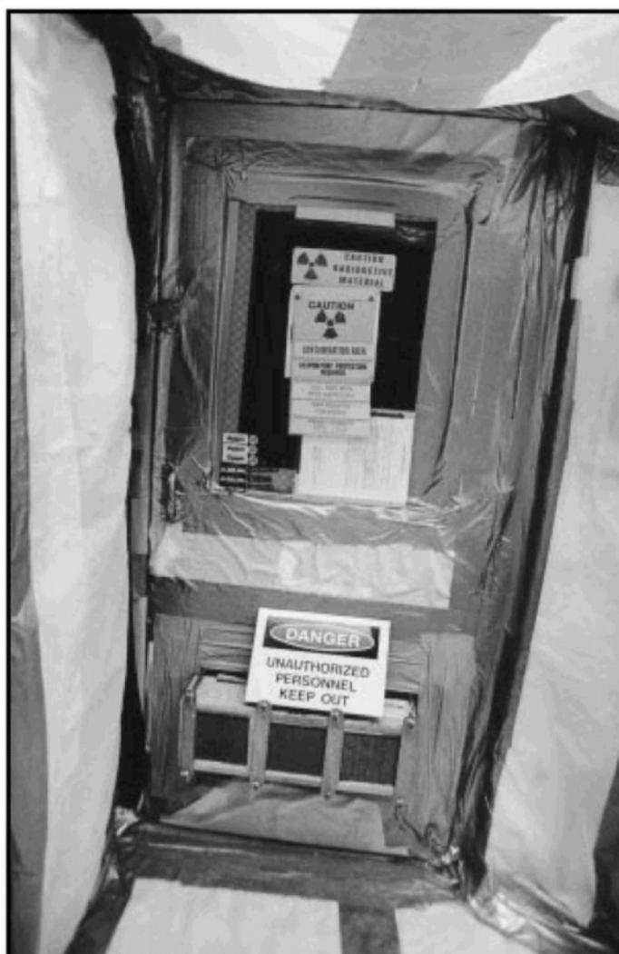
*FIGURE 2.6 Door leading into a plutonium processing room at the Rocky Flats Site is sealed due to very high levels of alpha radiation within the room. There are more than 20 such rooms at the site.
