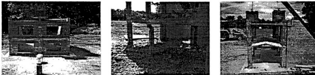
Figure 5: Exterior Wall With Window Opening, Severe Damage to Column and Floor
