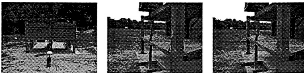
Figure 6: Solid Wall on Second Floor, Severe Floor and Column Damage
