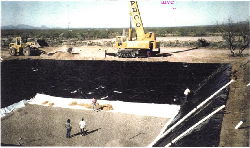
This photograph shows a lined basin constructed at the University of Arizona's Avra Valley Geophysical Test Site. The basin is 30 m by 30 m by 5 m deep. The entire basin was lined with high-density polyethylene; drain pipes were placed in the bottom and the basin refilled with native soil. This test site allows a closed system for injection and retrieval of fluids. During the summer of 1992, 24,170 liters of water were injected along a 1-m by 25-m strip at the center of the basin.
