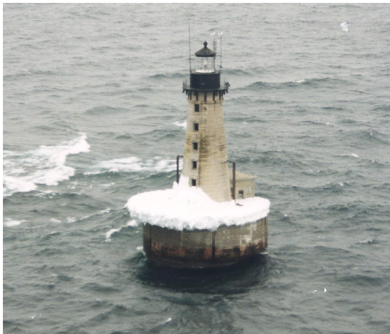
FIGURE 16 Pictures of representative C-MAN stations at Thomas Point, Maryland, and Stannard Rock, Michigan. (Source: U. S. Department of Commerce, National Oceanic and Atmospheric Administration)
