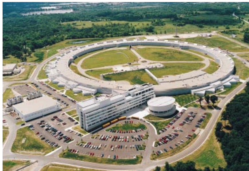
FIGURE 4.2 The Advanced Photon Source at Argonne National Laboratory, commissioned in 1996, is the nation's most powerful synchrotron x-ray facility. It will provide unprecedented research opportunities to thousands of users in the materials, biological, and engineering sciences. (Courtesy of Argonne National Laboratory.)
