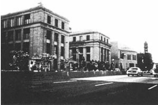
Figure 1. Existing 14th Street Side of the Bureau of Engraving and Printing.
