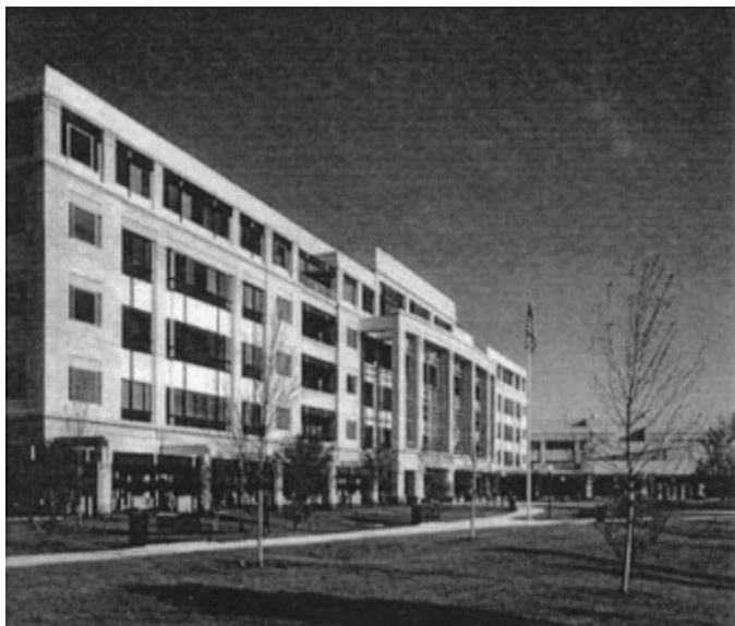
Figure 2. Facade of New HCFA Building.
