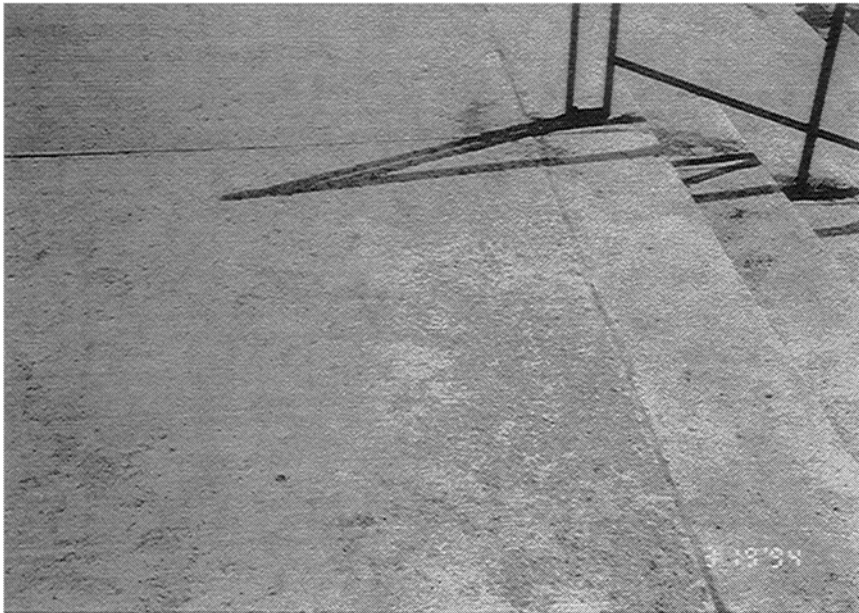
FIGURE 1–13 Salt scaling on concrete steps within six months of being cast caused by the use of deicing salts.
