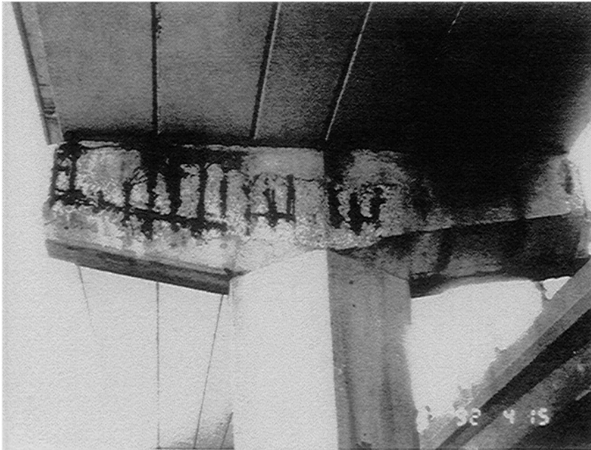
FIGURE 1–11 Corrosion of reinforcing steel in the support structure of an elevated highway caused by deicing salts seeping from the deck. The expansion of the corrosion products has caused spalling of the concrete cover. Source: Hansson, 1995.
