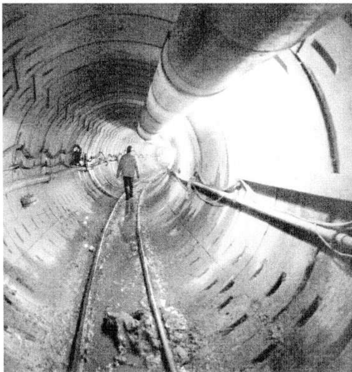
Figure 2 Soft-ground tunneling method used to control the inflow of water.
