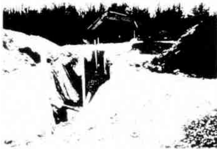
Construction of an infiltration trench for delivering fluids in an in situ bioremediation system. Courtesy of U.S. Environmental Protection Agency, R. S. Kerr Environmental Research Laboratory.
