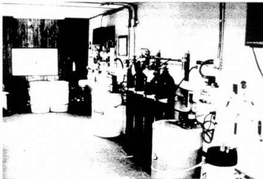
Equipment used to deliver nutrients and electron acceptors in an in situ bioremediation system. Courtesy of Ground Water Services, Houston, Texas.
