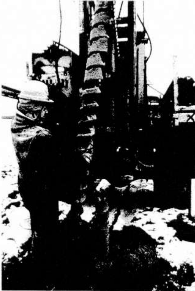
Hollow-stem auger used to obtain subsurface samples and install monitoring wells. Courtesy of U.S. Environmental Protection Agency, R. S. Kerr Environmental Research Laboratory.
