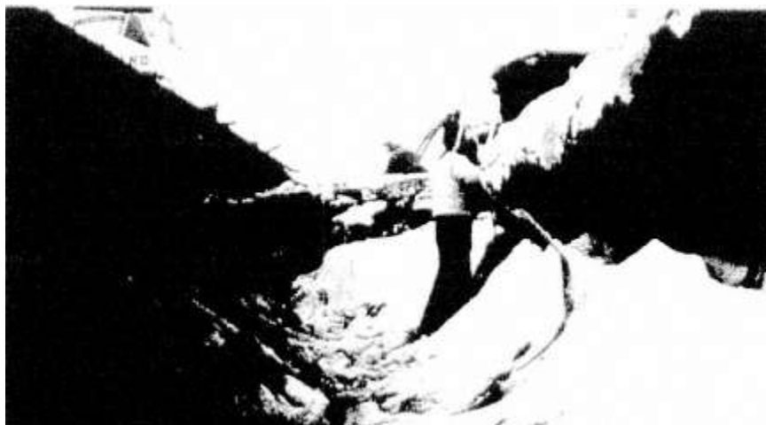
Excavating a trench during installation of piping for a ground water monitoring system. Courtesy of U.S. Environmental Protection Agency, R. S. Kerr Environmental Research Laboratory.
