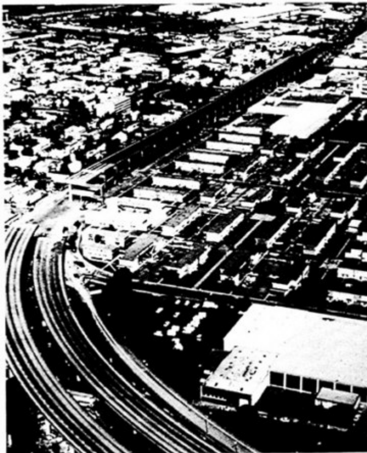
FIGURE 6-2 South section of Cypress Street Viaduct.
