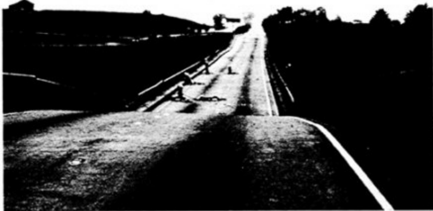
FIGURE 6-5 Collapsed Struve Slough Bridge.
