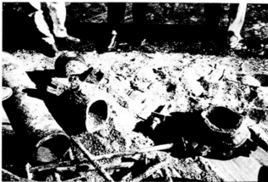
FIGURE 5-5 These specially designed cast-iron pipes were part of the AWSS in the South of Market area of San Francisco. Although there were few failures in this system, those that did occur had major impact on the fire-suppression water supply system.
