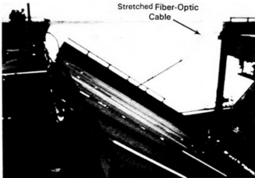
FIGURE 5-6 This photo shows a view of the collapsed upper deck of the Bay Bridge. Note in the background the fiber-optic cable that fell with the upper deck.
