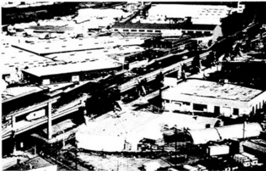
FIGURE 6-3 North section of Cypress Street Viaduct.
