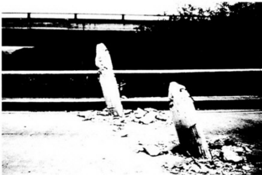
FIGURE 6-8 Piling penetrated six-inch deck between girder stems.
