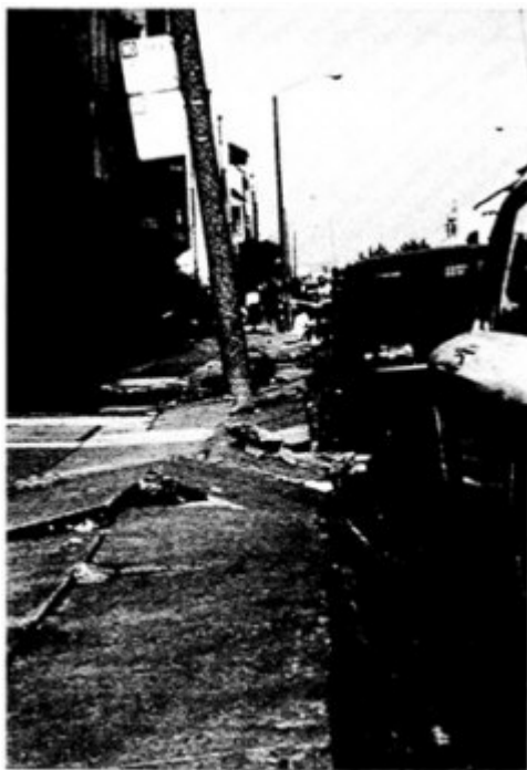
FIGURE 5.4 Extensive ground failure was observed in the Marina District of San Francisco. In addition to major damage to sidewalks and roadways, extensive damage to many of the underground utilities was observed.
