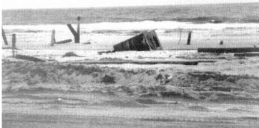
Figure 14-9 Exposed septic tank on Folly Island.
