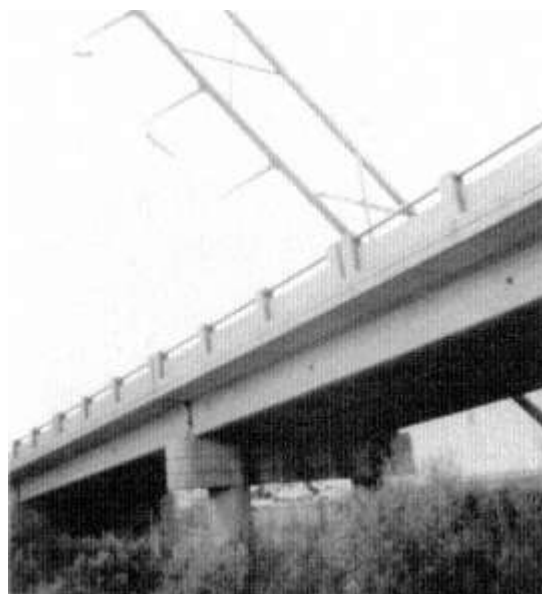
Figure 14-3 Timber transmission line support structure leaning against roadway in Charleston.
