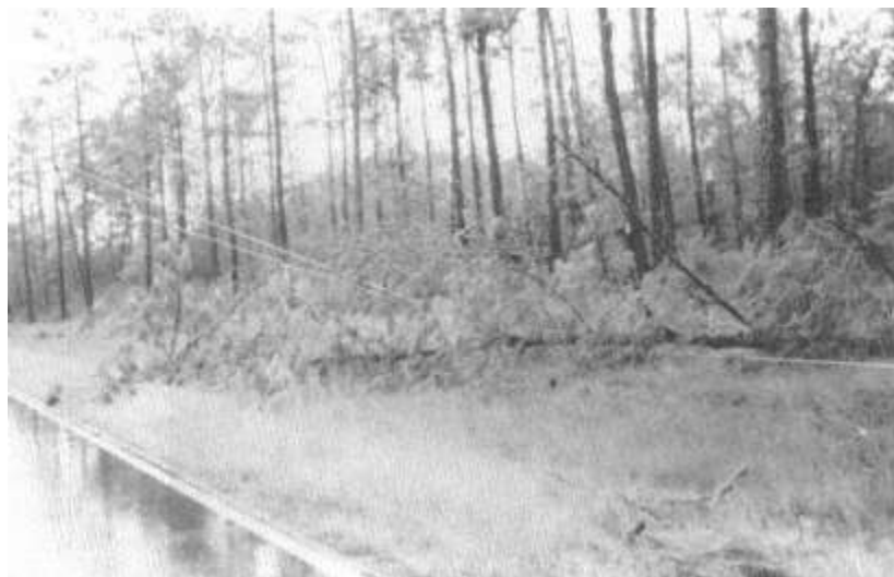
Figure 14-4 Distribution line downed by pine tree 60 mi inland.
