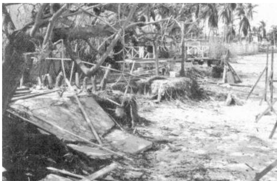
Figure 6-14 Punta las Marias area, same vicinity as Figure 6-13 , showing retreat of shoreline.
