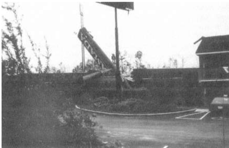
Figure 13-1 Typical damage associated with signs.
