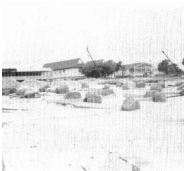
Figure 12-8 Shallow pier footings uprooted.
