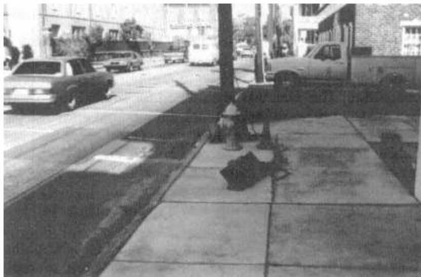
Figure 14-7 Traffic signal downed by wind.
