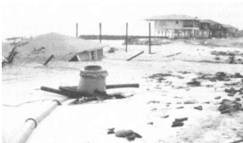
Figure 14-1 Destruction of roadway, electric lines, underground telephone lines, and water and sewer lines on the south end of Payleys Island.
