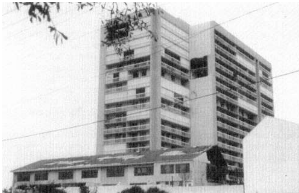
Figure 13-2 Typical damage to roofs.
