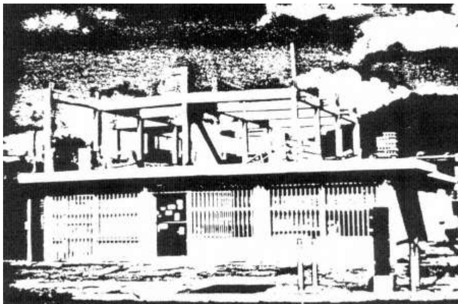
Figure 4-28 Reinforced concrete house under construction, Puerto Rico.
