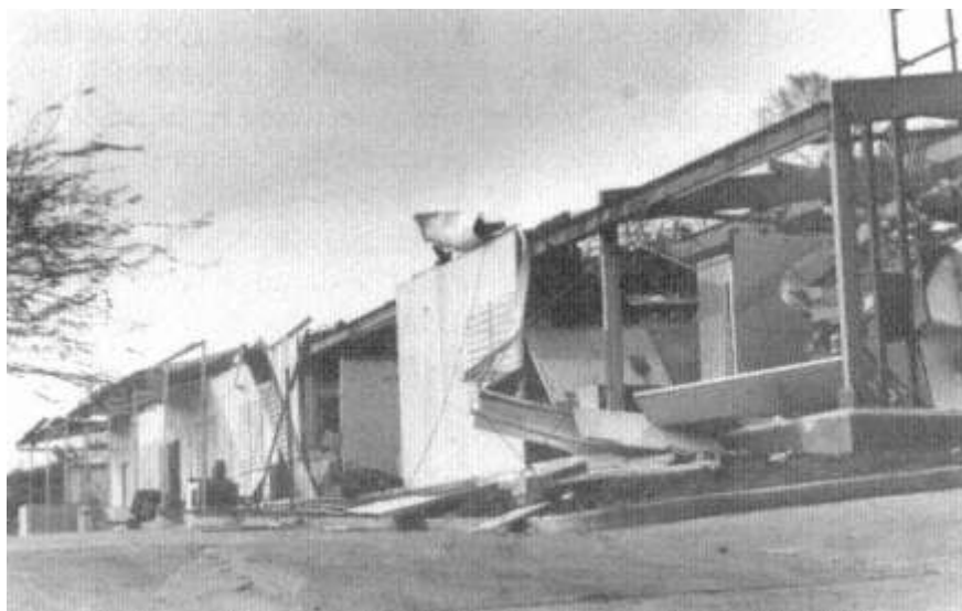
Figure 5-13 Damaged hospital at Culebra.
