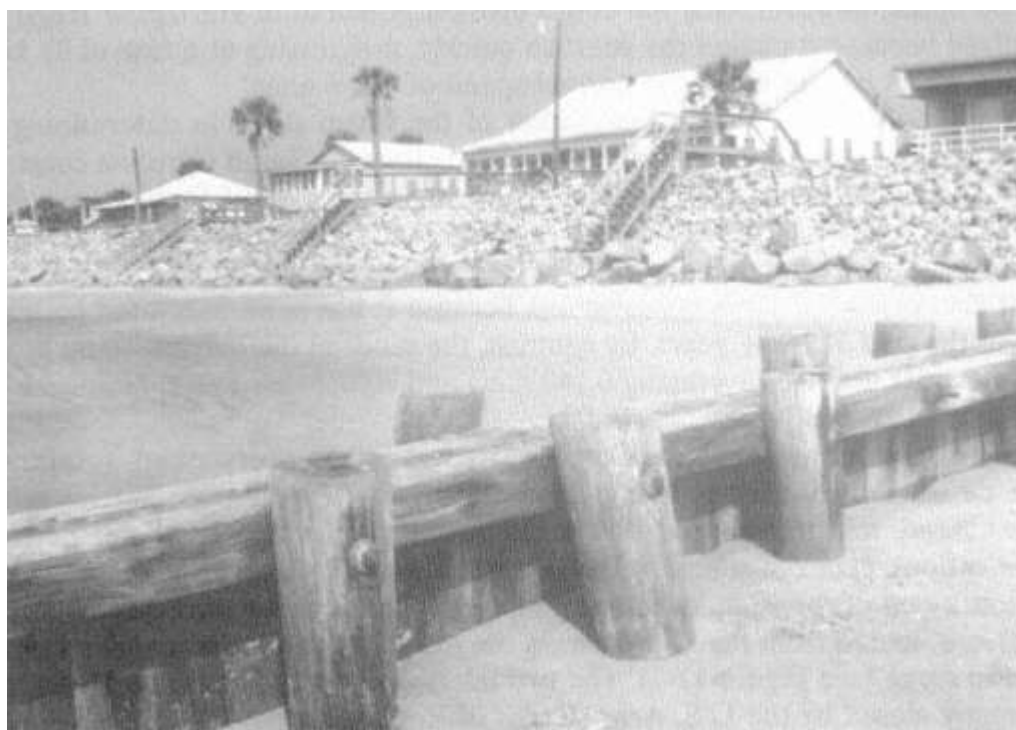
Figure 11-3 Pre-storm (July 1989) conditions at Folly Island, showing the limited dry beach area. Courtesy of Tony Pratt.
