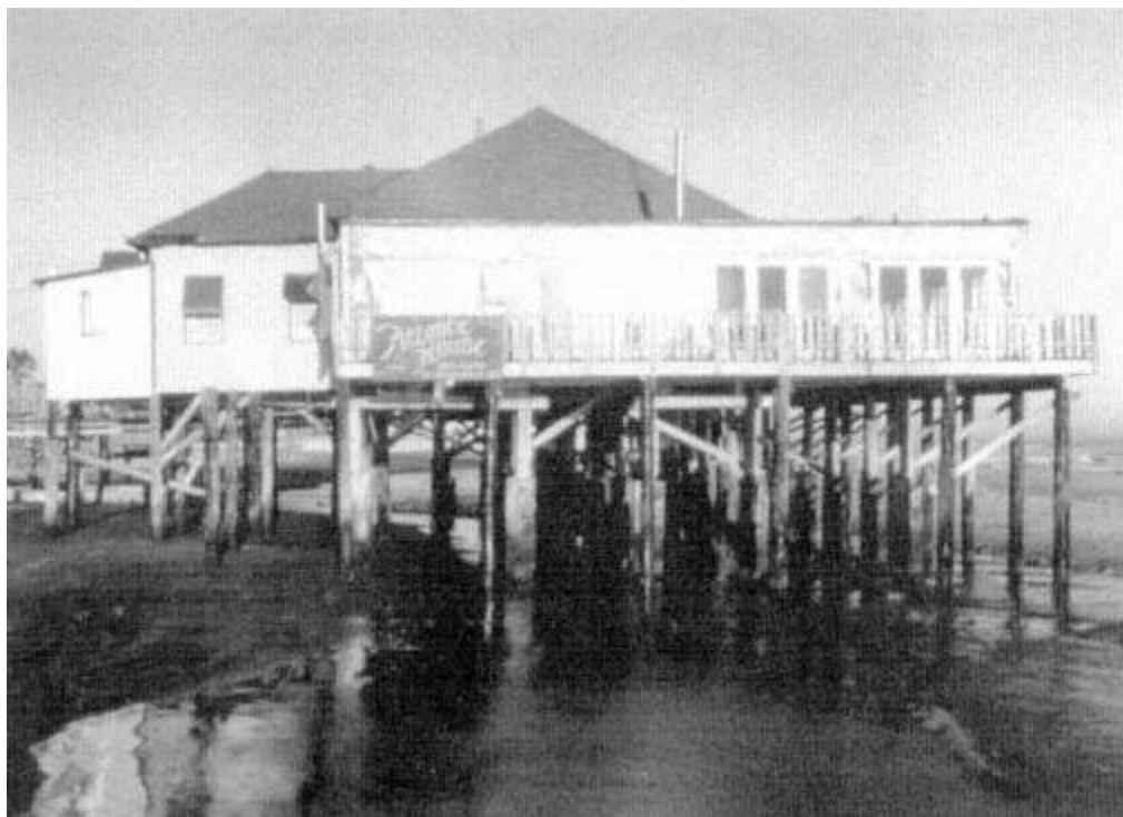
Figure 11-4a Pre-storm photograph of the Atlantic House restaurant.
