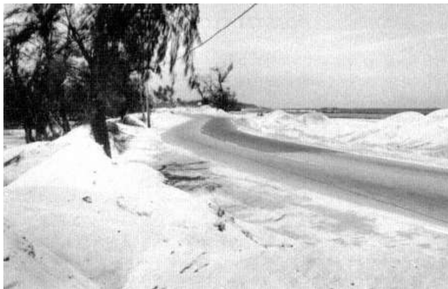
Figure 6-9 Overwash sand piled up along Route 187 in Pinones.
