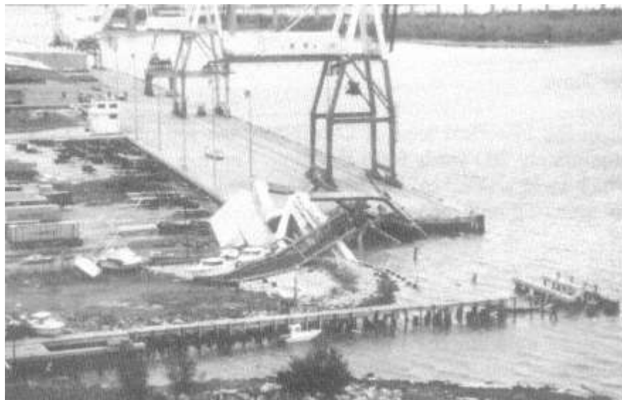
Figure 13-5 Damage to track-mounted cranes in industrial complex.
