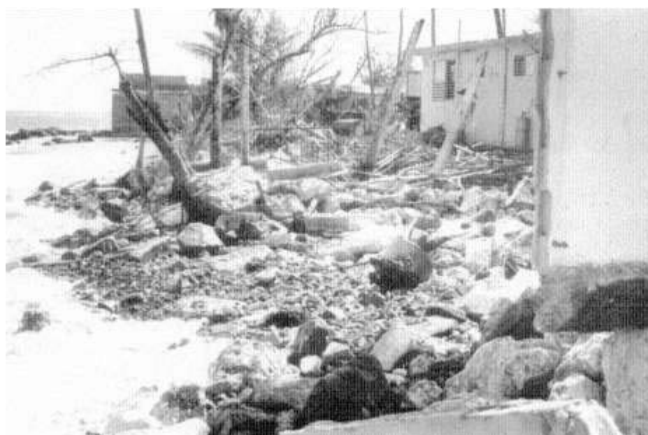
Figure 6-16 Punta Uvero area showing destruction of revetment and first row structures.
