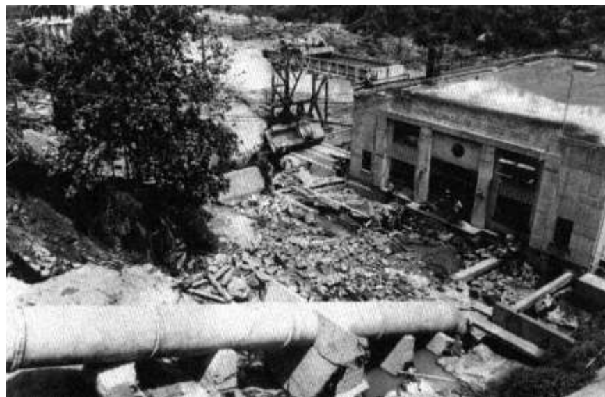
Figure 5-5 El Carraizo pumping plants, San Juan water supply.
