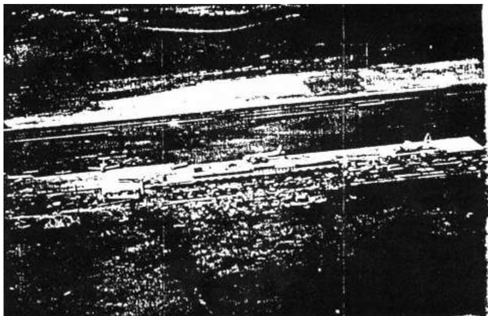
Figure 5-7 Alexander Hamilton Airport, St. Croix.
