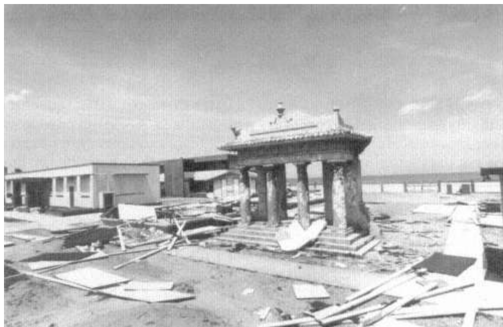
Figure 3-2b A second view of the Rosendo Matienzo Cintron School in Luquillo, Puerto Rico, used as a shelter during Hurricane Hugo.
