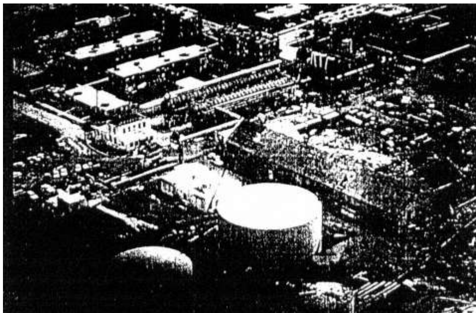
Figure 5-3 WAPA Richmond facilities, Christiansted, St. Croix.
