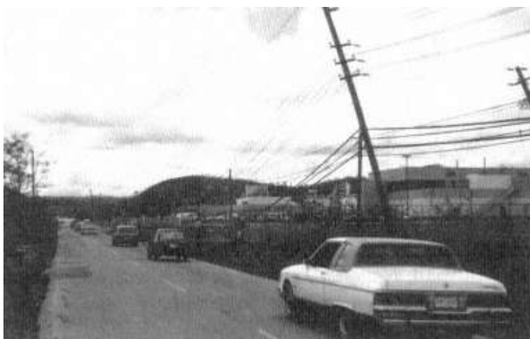
Figure 5-1 Downed power lines east of San Juan.
