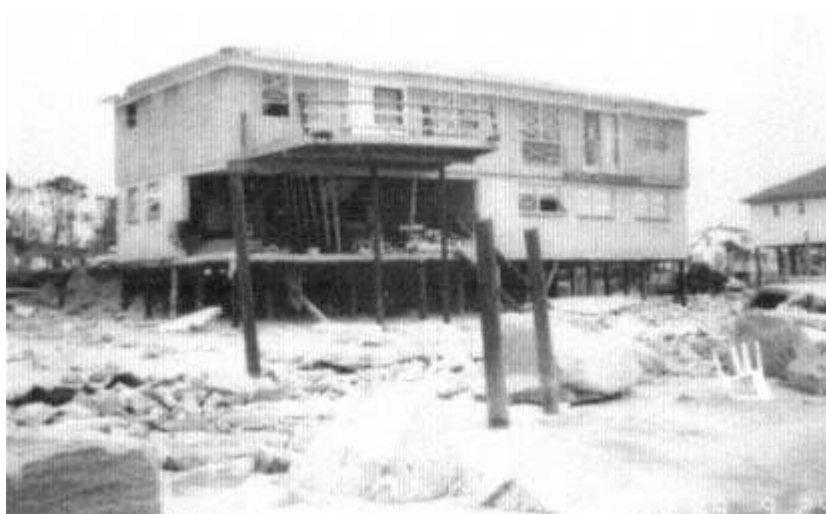
Figure 12-13b The access ramp washed into the house as a result of wave force.
