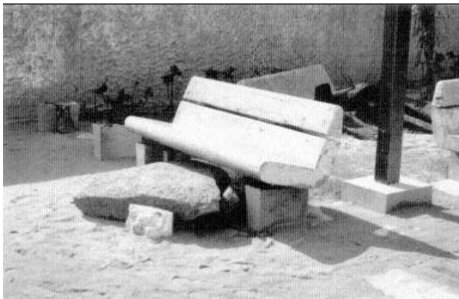
Figure 6-12 A boulder that had been thrown over a 1-m wall in the Condado. Site is immediately west of the Oasis Restaurant shown in Figure 6-11 .
