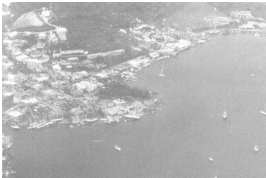
Figure 6-5 Ensenada Honda, the "hurricane proof" harbor of Culebra, showing ships grounded by storm surge. notice that ships did not float very far inland—testimony to the small penetration of storm surge owing to the steep terrain.
