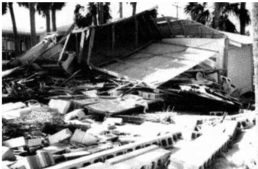
Figure 12-6 Structure with foundation on grade totally demolished by wave force.
