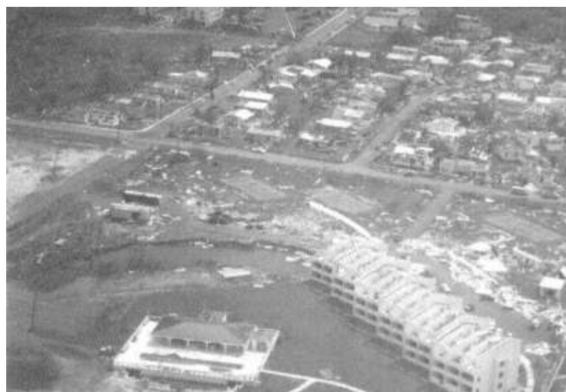
Figure 1-21d Microburst damage as seen from the low-flying aircraft over the north coast of St. Croix (second photo).
