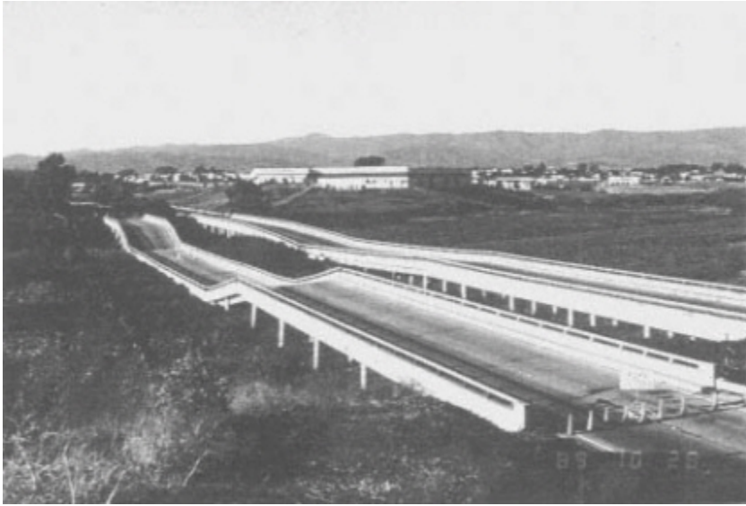
FIGURE 1-14 Collapsed bridge in Salinas River valley.
