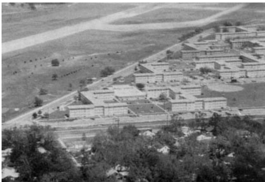
Figure 4-27 Reinforced masonry buildings at Keesler Air Force Base; roof damage caused leakage.
