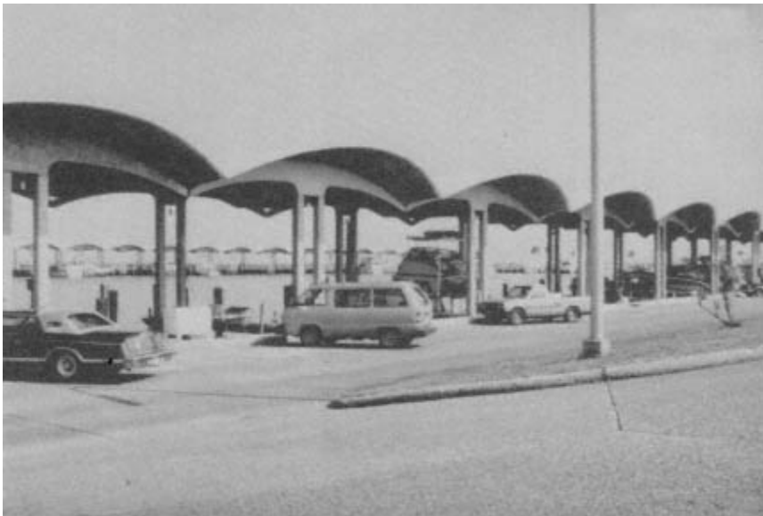
Figure 4-36 Broadwater-Beach Marina in Biloxi/Gulfport area. Precast concrete shelters sustained no damage.
