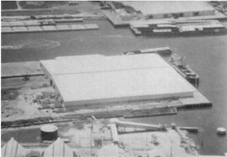
Figure 4-22 Preengineered warehouse buildings at Ingalls Shipyard. Wind damage limited to older building (top).
