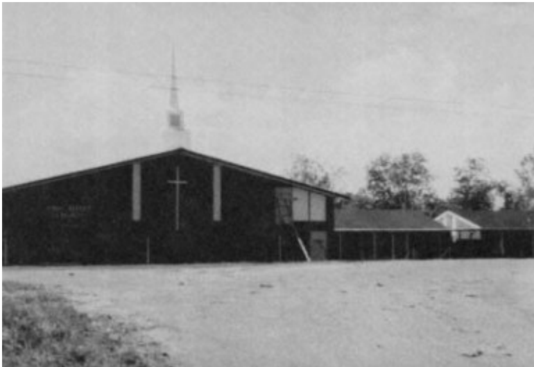
Figure 4-25 First Baptist Church of Lyman. Wind damage to complex of metal buildings limited to glass breakage due to windborne debris.
