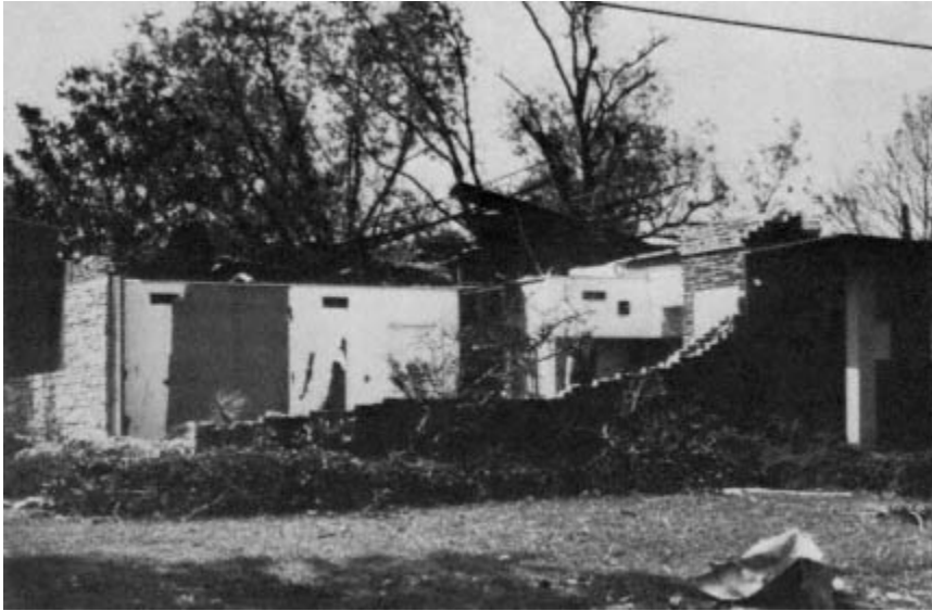
Figure 4-14 Damaged house using metal deck roof, Pascagoula.
