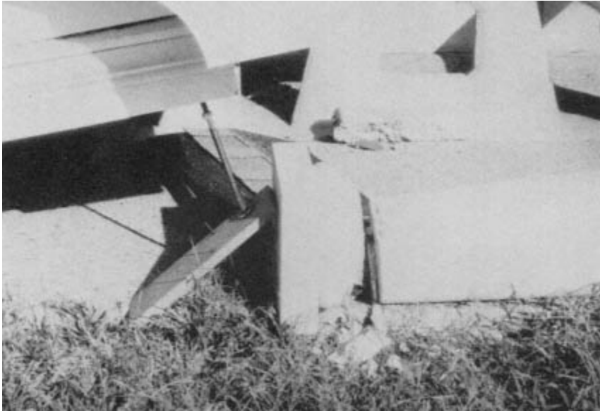
Figure 4-33 Column-to-roof connection of shelter of Figure 4-31 .
