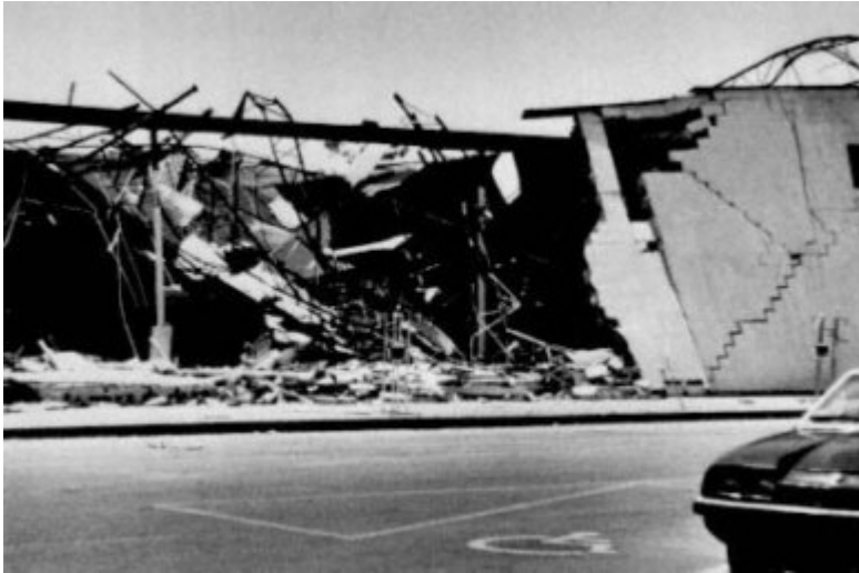
Figure 4-4 Detail of roof and wall damage in Figure 4-3.
