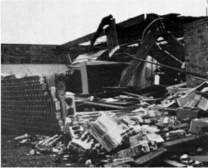
Figure 4-7 Collapse of Payless Shoe Store, Pascagoula.
