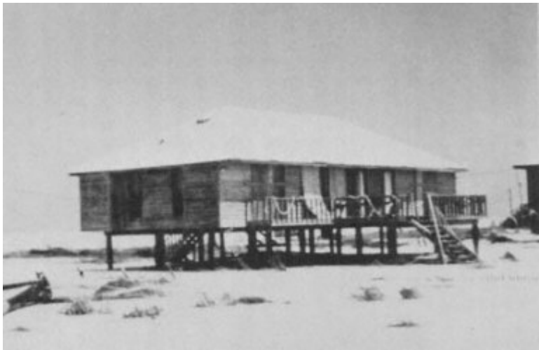
Figure 4-40 Undamaged older beach house with steep-pitched roof and protected windows, Dauphin Island.
