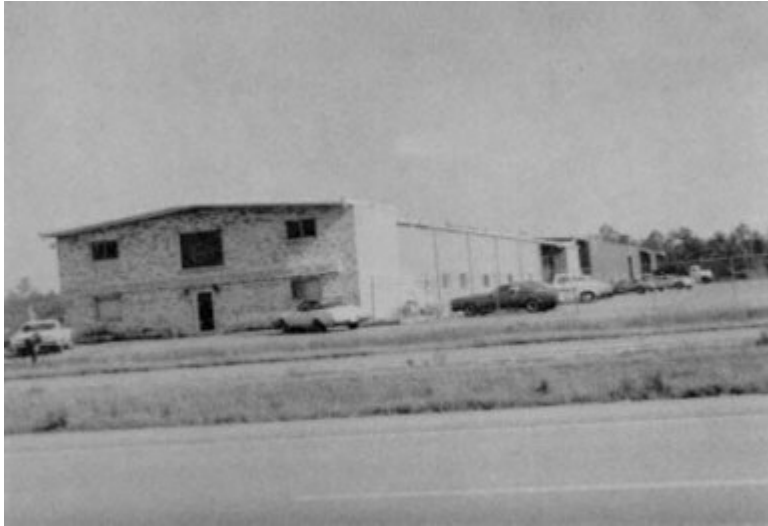
Figure C-5 Metal building clad with masonry veneer located in Gautier.
