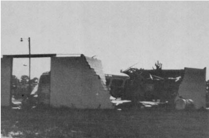
Figure 4-11 Collapse of masonry-walled garage following loss of roof, Pascagoula.
