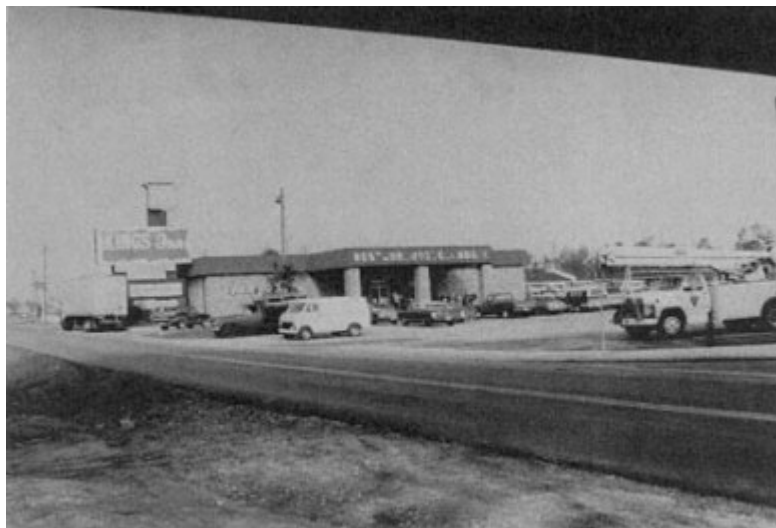
Figure 4-26 Preengineered metal building in Pascagoula. Wind damage limited to logo.
