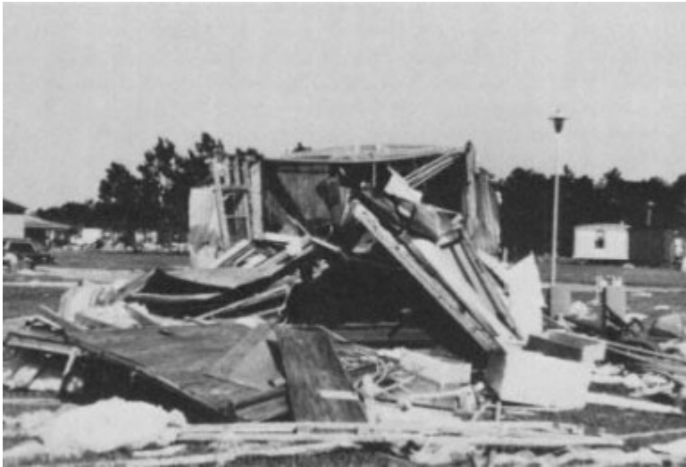
Figure 4-19 Structural damage to well-anchored mobile home, Gautier.
