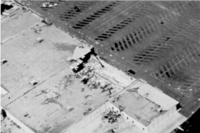
Figure 4-3 Collapse of a section of the Jackson Square Shopping Center, Gautier.
