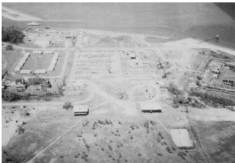
Figure 4-47 Fort Gaines area showing damage to flat-roofed buildings, Dauphin Island.
