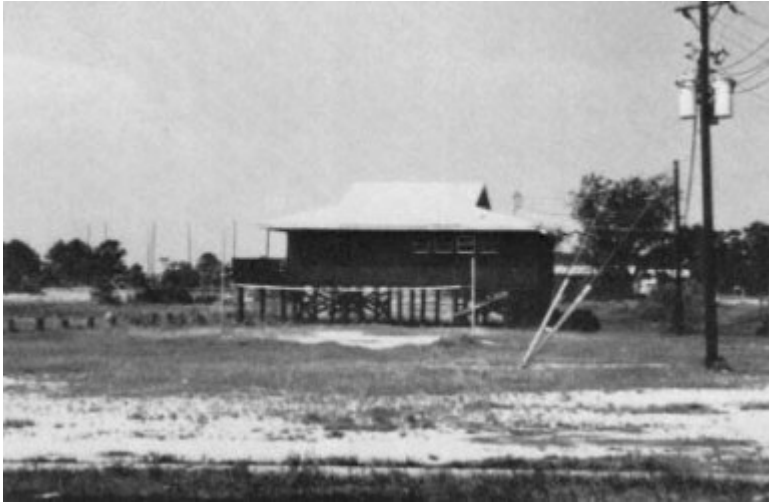
Figure 4-39 Well-constructed modern building, near Fort Gaines, Dauphin Island.
