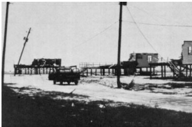
Figure 4-43 Repeated damage patterns in similarly constructed buildings, Dauphin Island.
