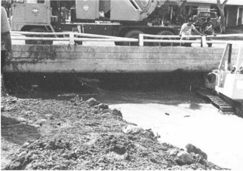
Figure 18a Bridge over east fork of Niu stream at Halemaumau Street.
