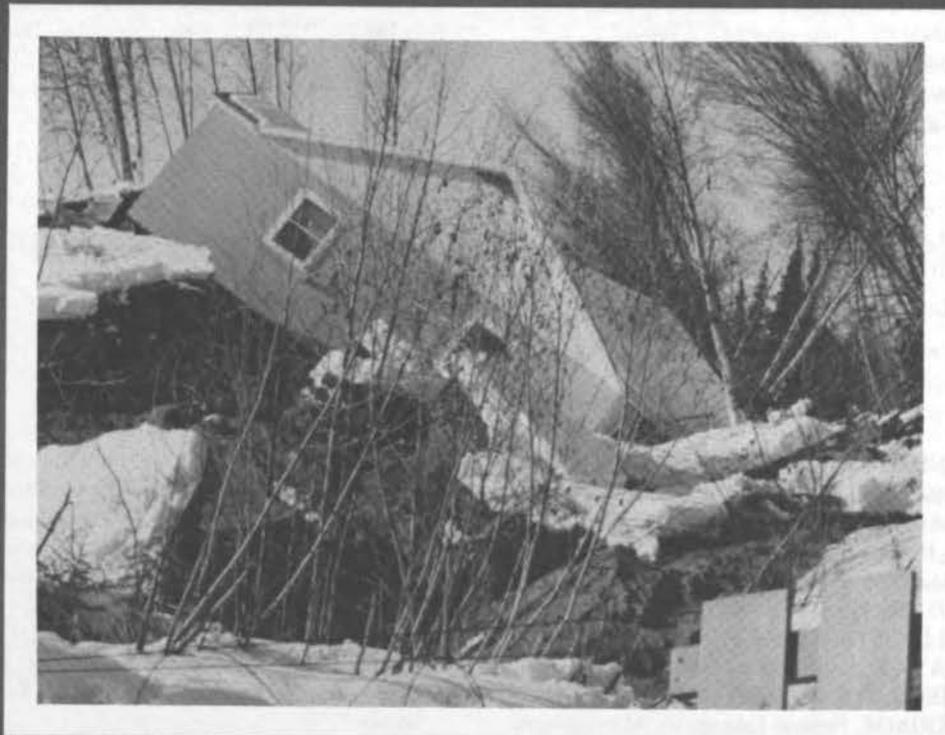
*Earthquakes often trigger massive landslides, such as the one shown here in the Turnagain Heights subdivision in Anchorage, Alaska. The great Alaskan earthquake of March 1964 (magnitude 8.4), liquified sand lenses beneath the subdivision, causing a complex slide with severe surface contortion. During the four minutes of perceptible ground shaking, the front of the slide moved more than 1,000 ft, destroying 35 homes. (Source: G. W. Housner, California Institute of Technology.)*
