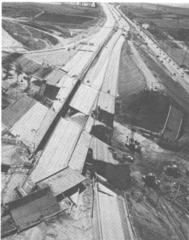
*On February 9, 1971, the magnitude 6.5 San Fernando, California, earthquake damaged 42 freeway bridges and collapsed five, including these in the Sylmar region of Los Angeles. Since then, California highway officials have required overpass designs to incorporate dynamic analyses and the results of extensive earthquake engineering research. (Source: G. W. Housner, California Institute of Technology.)*
