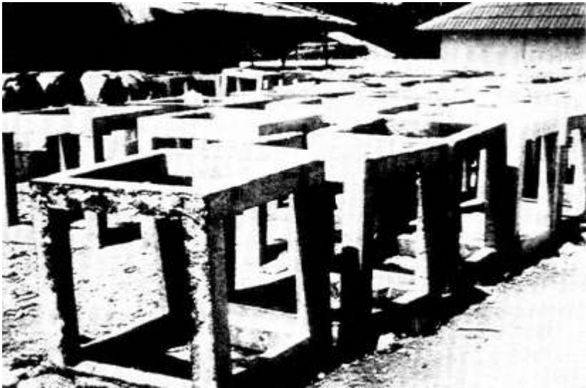
Figure 3.11 Concrete cubes are fabricated for an artificial reef in the Andaman Sea, Thailand. (J. J. Polovina)
