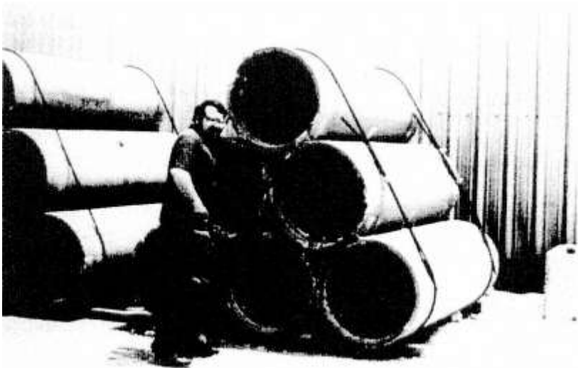
Figure 3.10 Damaged drainage pipes are widely used as artificial reefs. (D. Feigenbaum)
