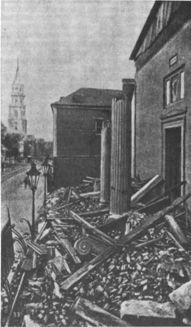
FIGURE 2 Photograph of building collapse in Charleston, South Carolina. This destructive earthquake occurred August 31, 1886 and caused considerable damage. Its estimated magnitude was 7.7. Source: Dutton (1890).
