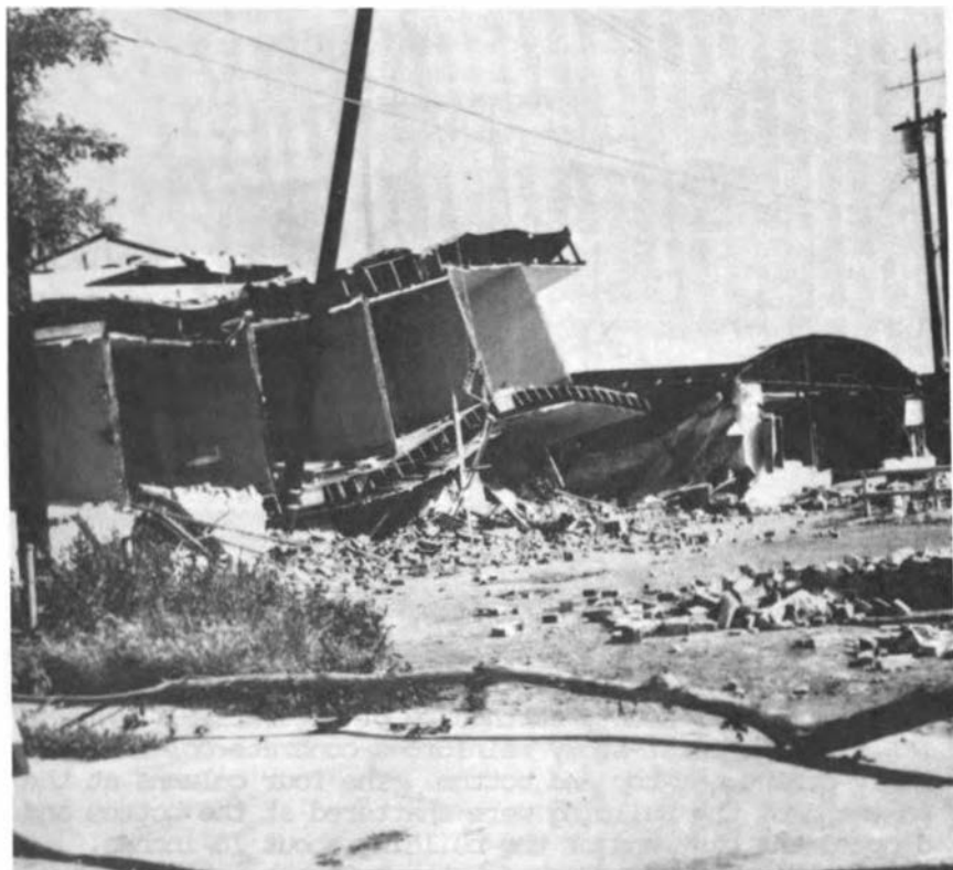
FIGURE 13 Structural damage to a brick building resulting from the Coalinga earthquake of May 2, 1983. The epicenter of this magnitude 6.5 shock was about 10 miles from the town. Such buildings, not designed to resist earthquakes, are very vulnerable to damage. Source: California Division of Mines and Geology (1983). (Photograph by James Stratta)
