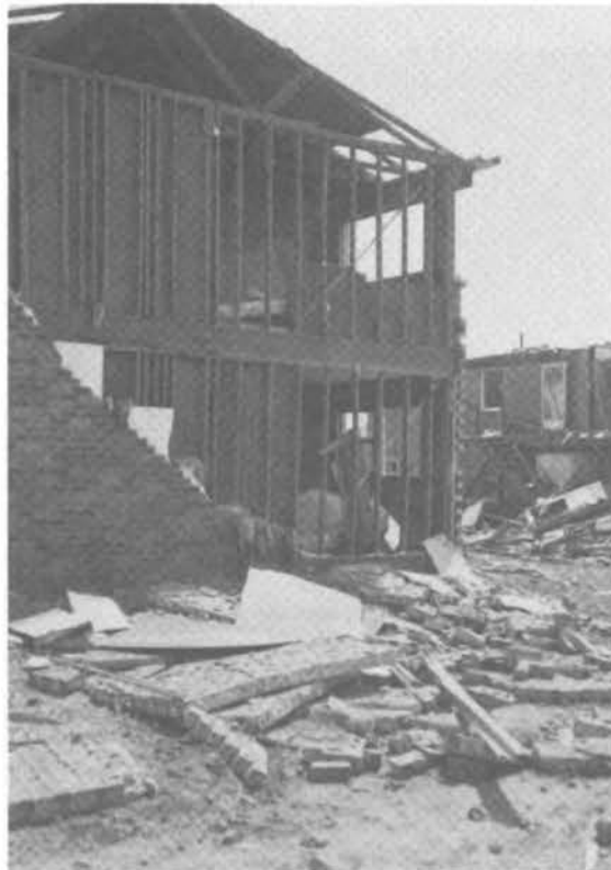
FIGURE 15 Detail of Hillcrest Apartments showing lack of continuity of plywood sheathing.
