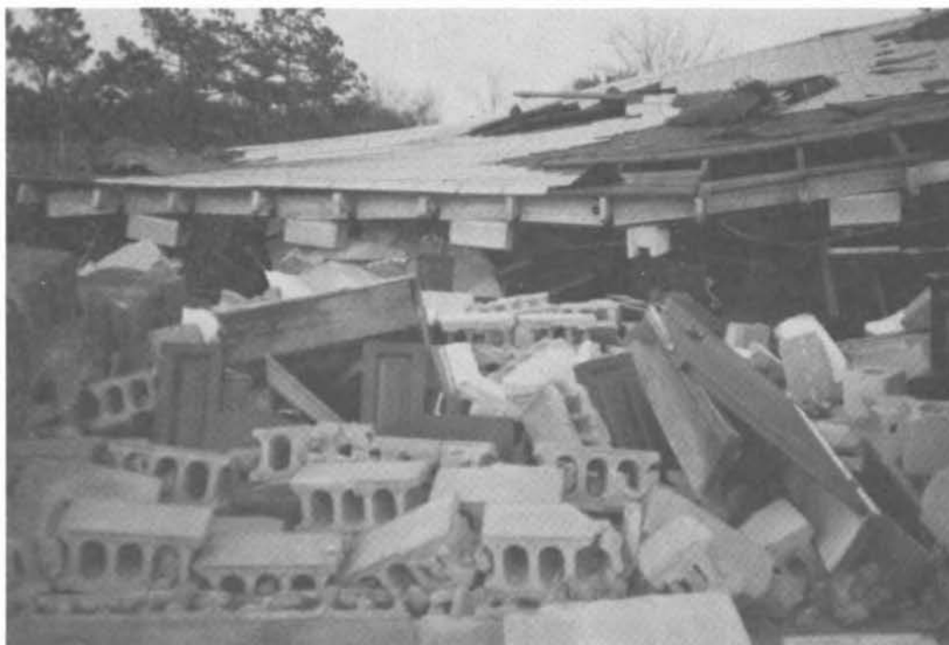
FIGURE 27 Detail of church showing roof-wall connection.
