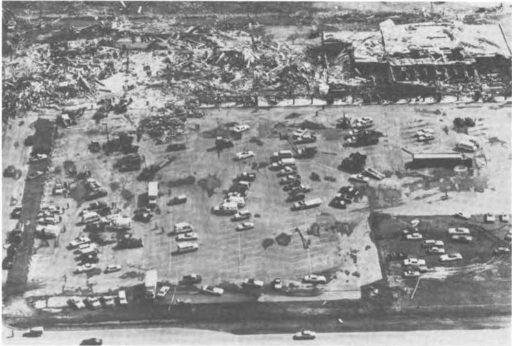
FIGURE 35 Aerial view of damage to Northwood Village Shopping Center. (Photograph courtesy The State. )
