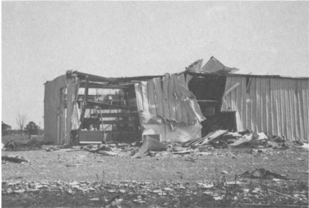
FIGURE 32 Steel-framed retail store in Bennettsville.
