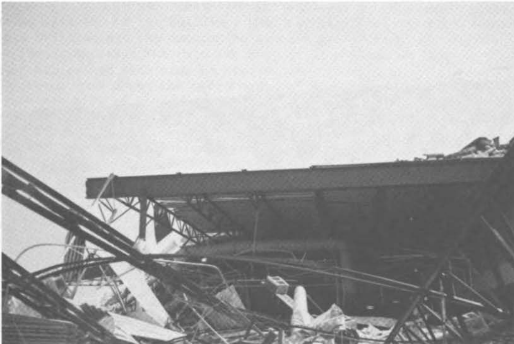
FIGURE 38 Failure of beam joint.
