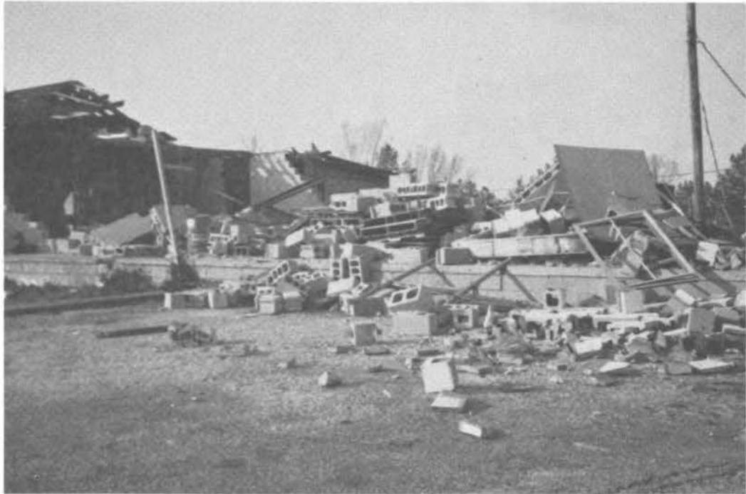
FIGURE 22 Masonry retail store in Winnsboro.
