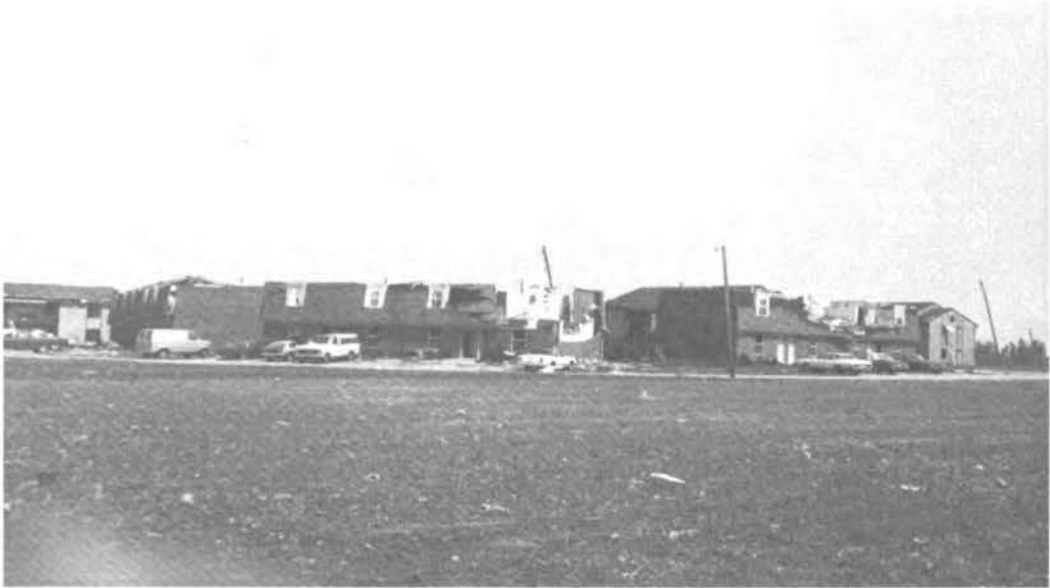
FIGURE 13 Marlboro Court Apartments in Bennettsville.
