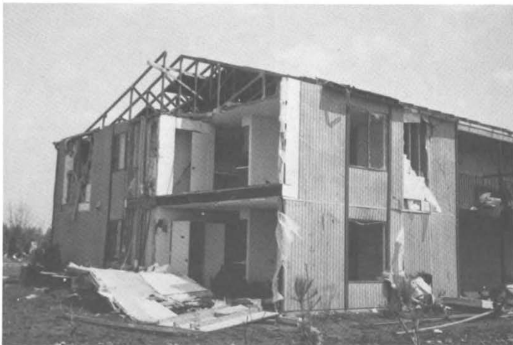
FIGURE 18 Detail of Marlboro Court Apartments showing continuity provided by wood siding.
