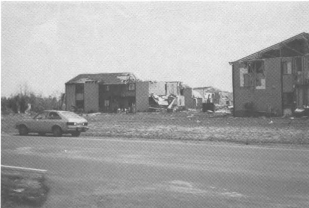
FIGURE 12 Marlboro Court Apartments in Bennettsville.
