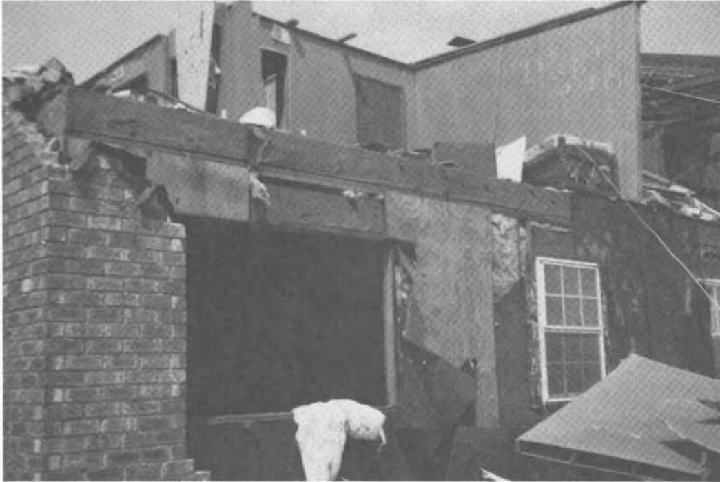
FIGURE 15 Detail of Hillcrest Apartments showing lack of continuity of plywood sheathing.
