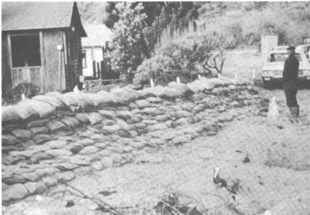
FIGURE 70 Sandbag barrier at Stinson Beach to prevent flooding from waves and sand deposition from overwash.
