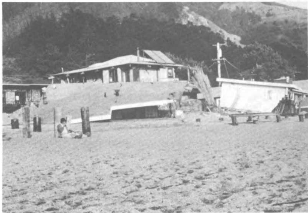
FIGURE 68 Dwellings damaged in Stinson Beach due to erosion undermining and direct action of waves.
