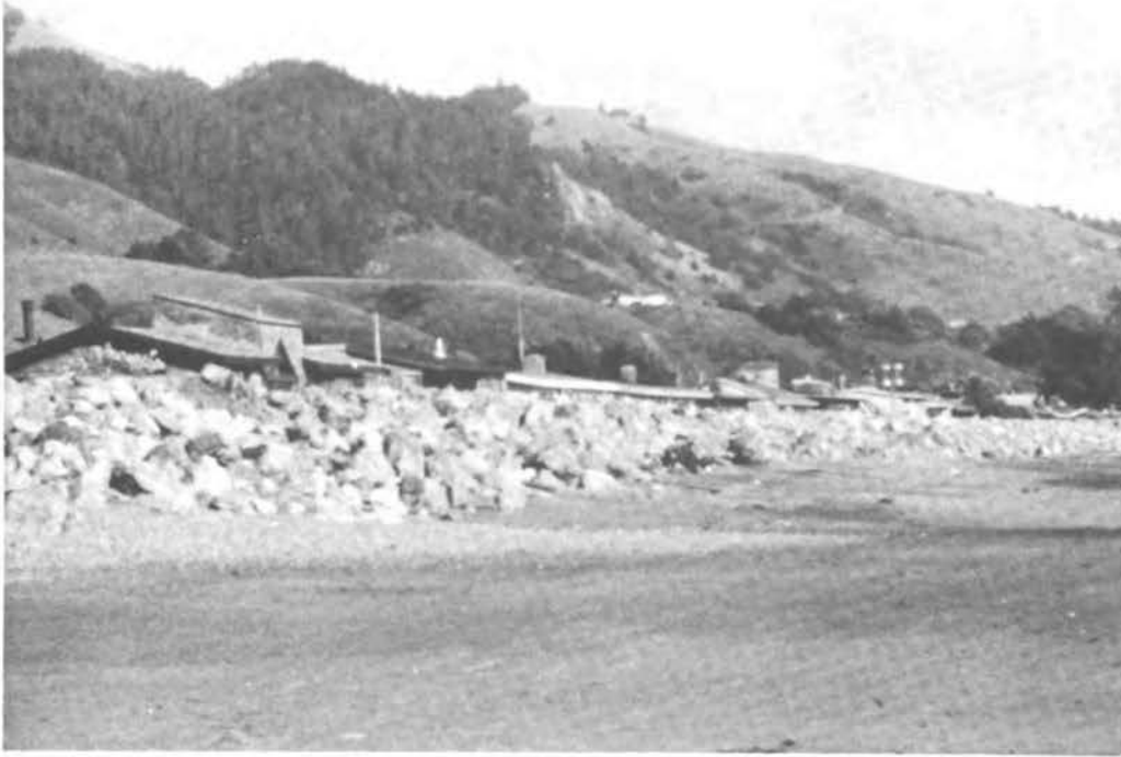
FIGURE 65 Substantial revetment in Stinson Beach to protect dwellings from erosion and waves.
