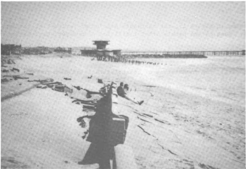
FIGURE 16 This structure supported by light piles escaped direct wave damage. The Venice Pier is in the background.
