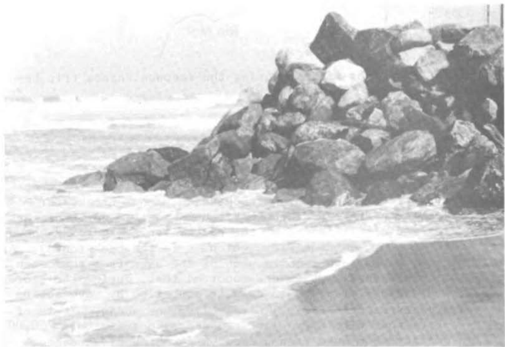
FIGURE 26 Closeup of revetment shown in Figure 25.
