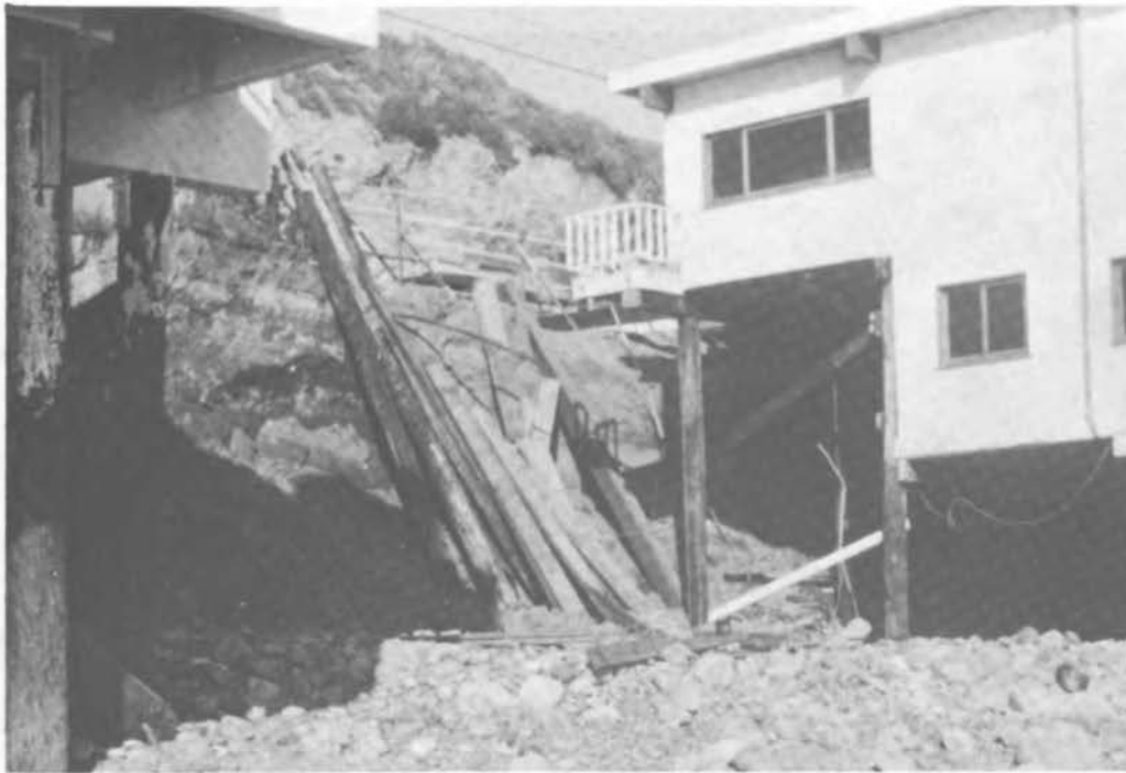
FIGURE 44 Location where a dwelling in Malibu Beach was destroyed by waves. Most of the debris had been removed at the time of this photograph.
