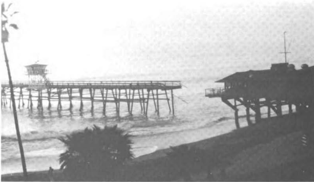
FIGURE 14 Nearshore section of the San Clemente Pier removed by storm.
