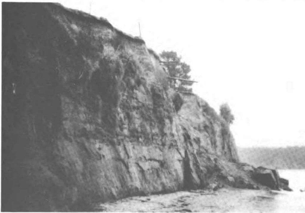
FIGURE 72 Failure of coastal cliff at Capitola.
