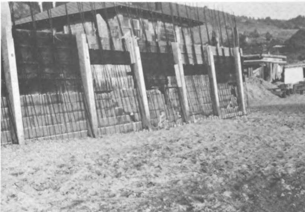
FIGURE 66 Reinforced concrete seawall in Stinson Beach being constructed.
