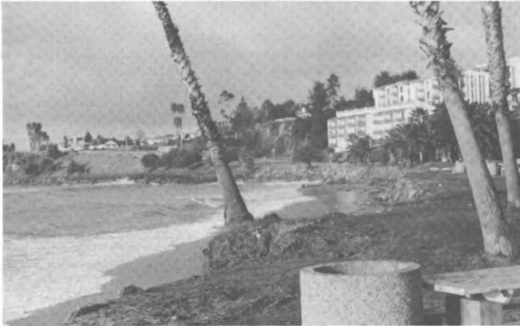
FIGURE 51 View west from west end of Leadbetter Beach. The beach and upland were substantially eroded, with the loss of a number of palm trees.
