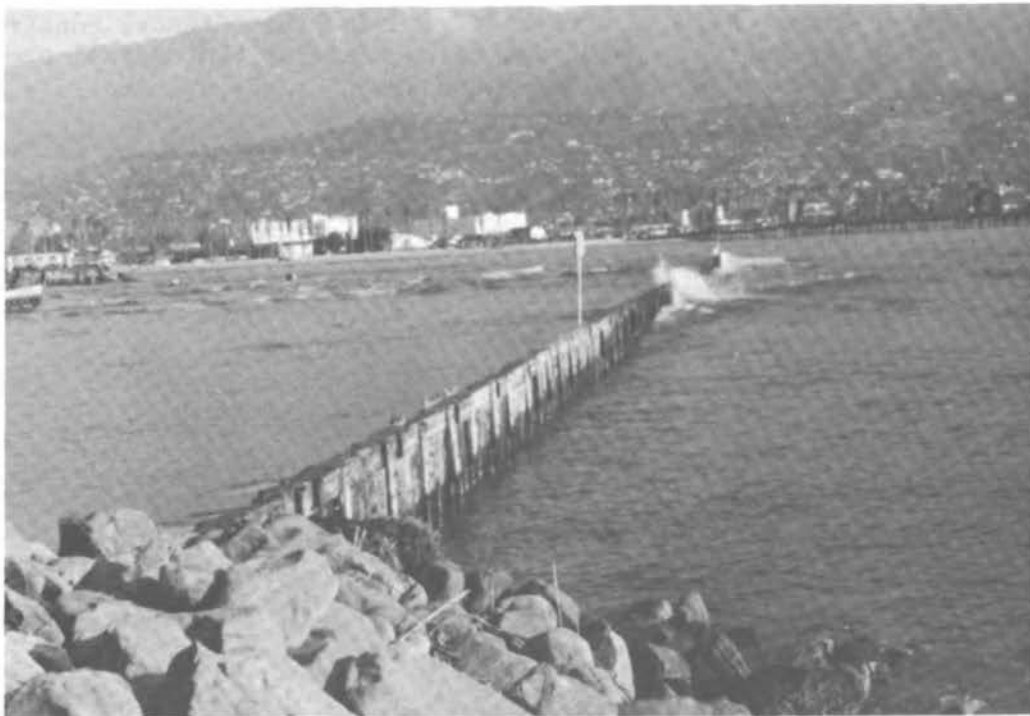
FIGURE 52 View looking north from the base of the timber sheet-pile structure that extends north from the Santa Barbara breakwater.
