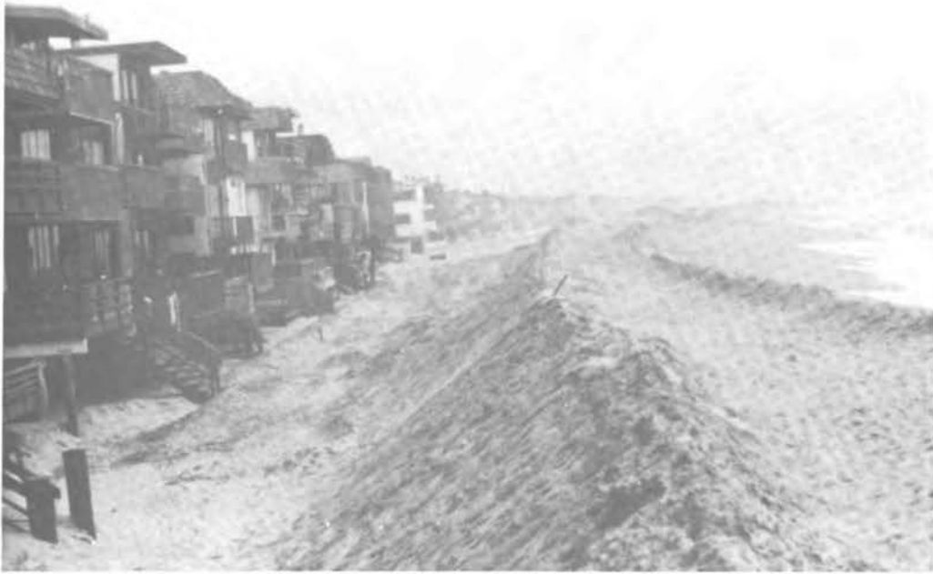
FIGURE 37 A sand berm overlies revetment as protection against flooding at Surfside Colony.
