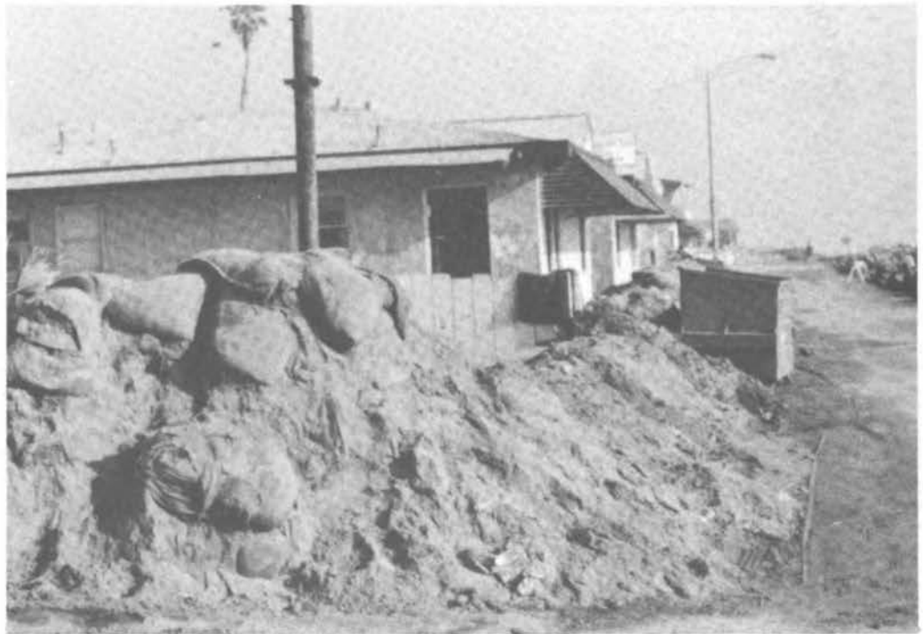
FIGURE 30 Oceanside Beach showing efforts to protect oceanfront cottages against water and debris damage.
