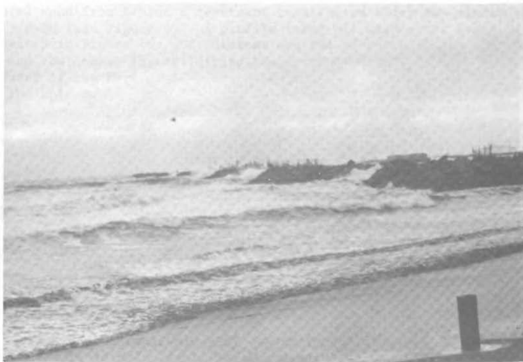
FIGURE 38 The south jetty at the entrance to Anaheim Bay.
