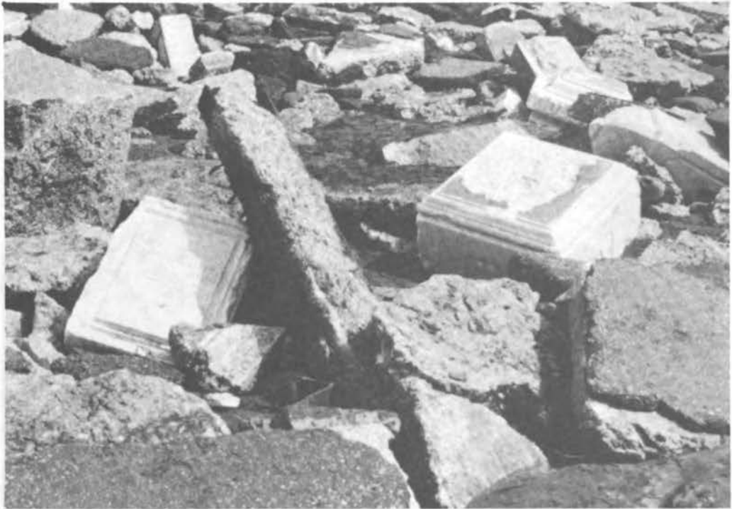
FIGURE 63 Makeshift revetment for road protection at Ocean Beach including headstones from cemetery.
