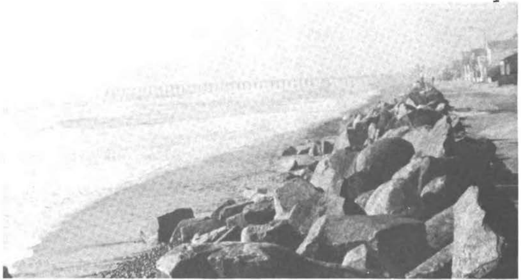
FIGURE 29 Oceanside Beach with Oceanside Pier in the background. Note the narrow beach, revetment, and evidence of overtopping.
