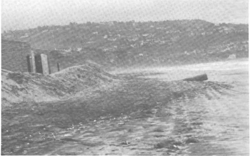
FIGURE 39 Torrance County Beach. Severe erosion is threatening the restroom facilities. Heavy minerals (black sand) were left as "lag" deposits on the beach. The Palos Verdes Hills are in the background.
