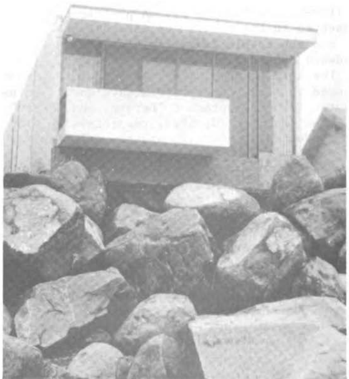
FIGURE 42 Heavy revetment fronting a dwelling in Malibu Beach.
