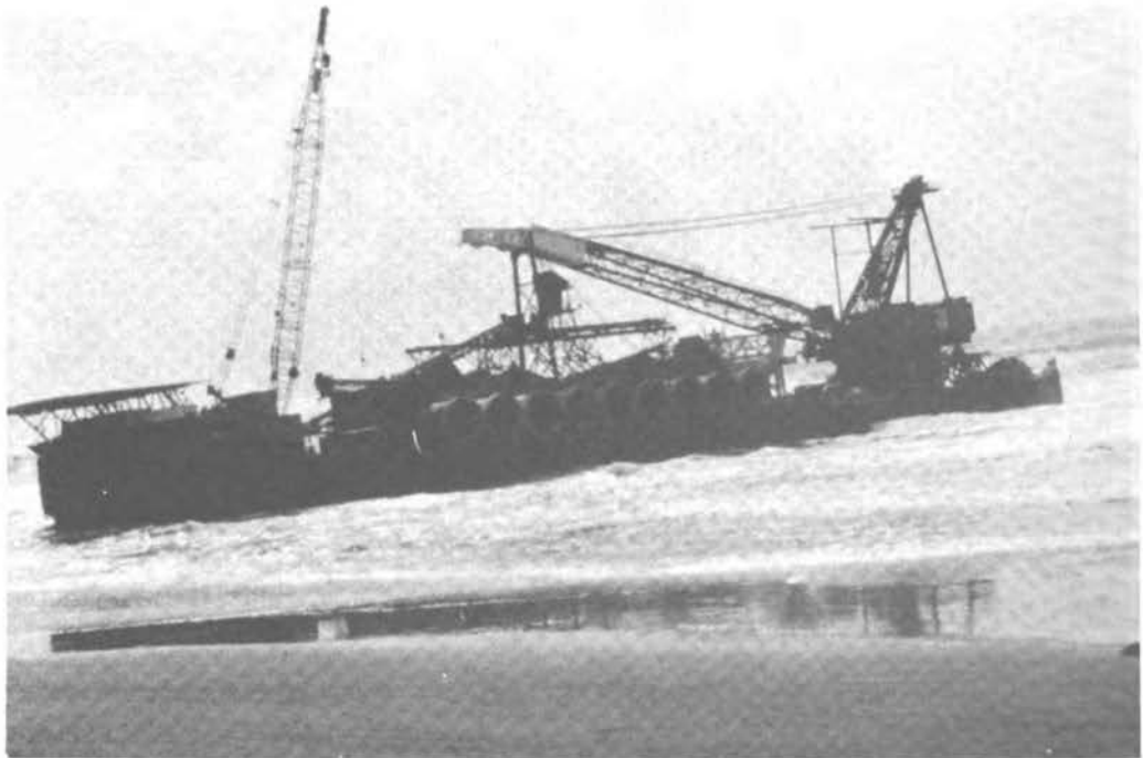
FIGURE 64 The stranded construction barge Betty L at Ocean Beach with efforts under way to free this casualty of the storm.
