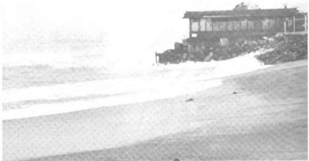
FIGURE 25 View of Imperial Beach showing eroded beach and home protected by revetment (photograph was taken at low tide).
