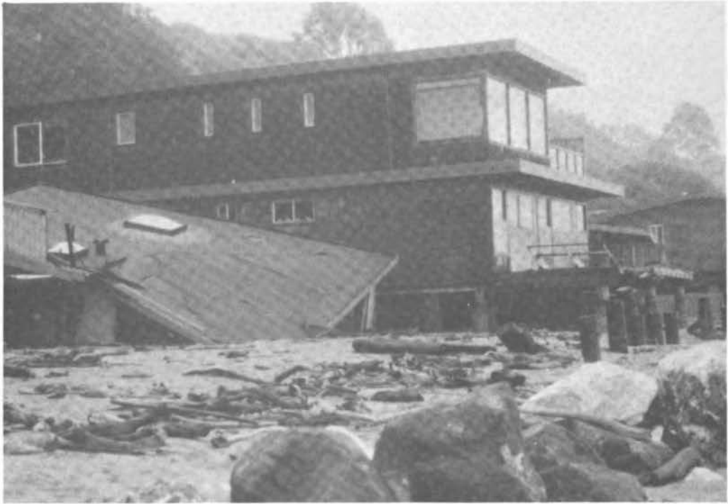
FIGURE 55 Destroyed home in Rio Del Mar Beach. Note the ineffective revetment fronting the structure.
