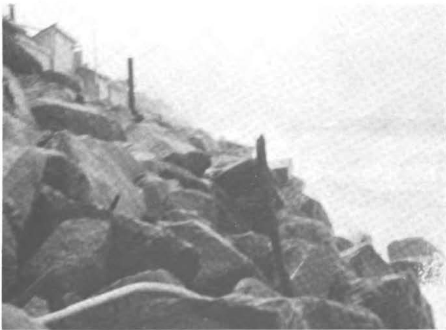
FIGURE 54 Heavy revetment protecting upland structures in Rio Del Mar Beach.
