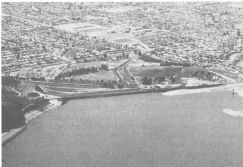
This photograph of the Lower San Fernando Dam, taken a week after the 1971 earthquake, shows the extensive residential area below the dam. Eighty thousand residents were evacuated for three days until the reservoir was lowered to a safe level.
