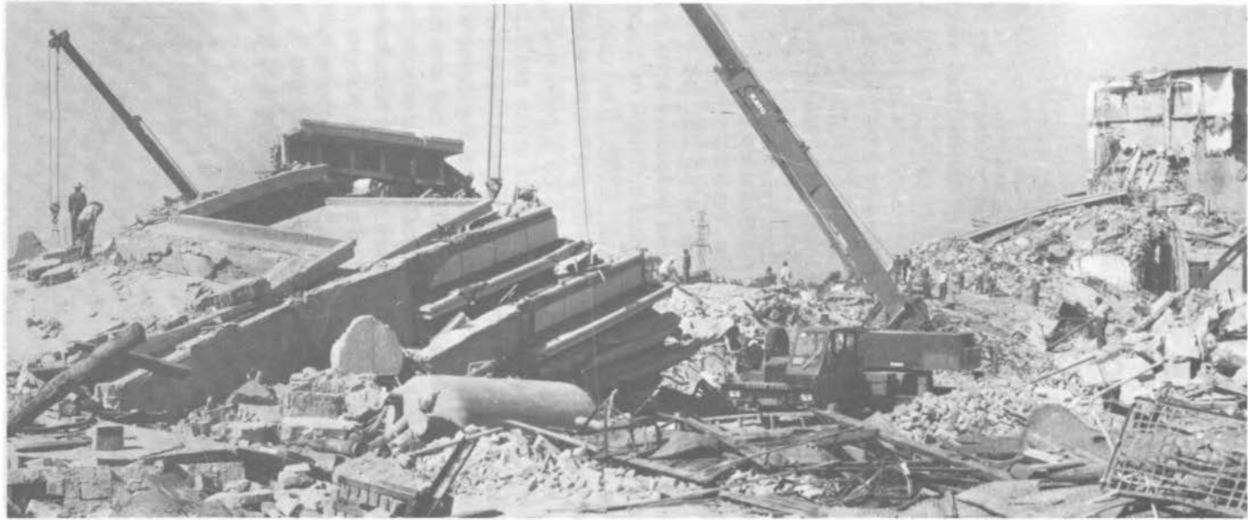
This hospital building in the city of Tangshan, China, collapsed after the earthquake of July 28, 1976. A magnitude 7.8 earthquake centered under this industrial city of one million people created one of the greatest earthquake disasters in history. Eighty five percent of the buildings either collapsed or were severely damaged, and several hundred thousand people were killed. Earthquake-resistant design was not required by the building code, so the city was almost completely unprepared. A visit to the city in September 1982 revealed that a strenuous rebuilding effort was under way. The other 39 provinces had been called upon to provide engineering, architectural, and construction services and materials. Reportedly, four years after the earthquake a sufficient number of apartment houses had been constructed to accommodate about half the population.
