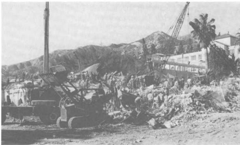
The Sylmar Veterans Administration Hospital collapsed during the 1971 San Fernando, California, earthquake. Forty-nine people were killed in the collapse, and 16 survivors were dug out of the ruins. This photograph was taken 2-1/2 days after the earthquake, just before the last survivor was found.
