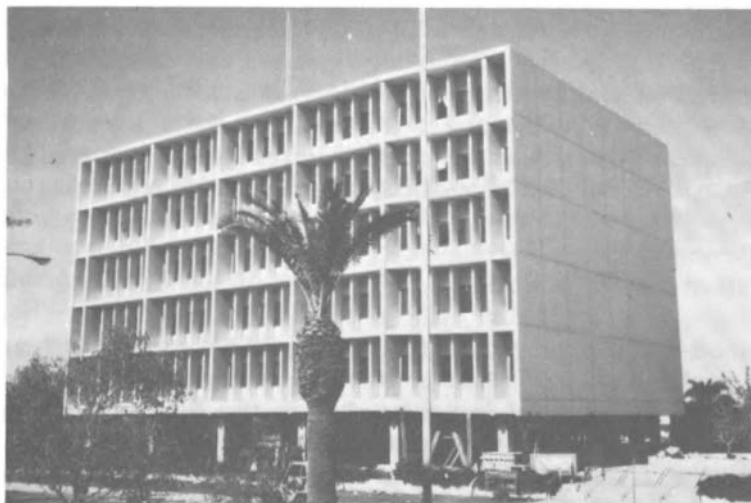
The Imperial County Services building was severely damaged by the 1979 magnitude 6.4 Imperial Valley, California, earthquake. The building, designed in 1968, was located 7 miles from the fault. The motions of the building and the ground during the earthquake were recorded, giving engineers records of motions for the first time from a building undergoing severe structural damage.
