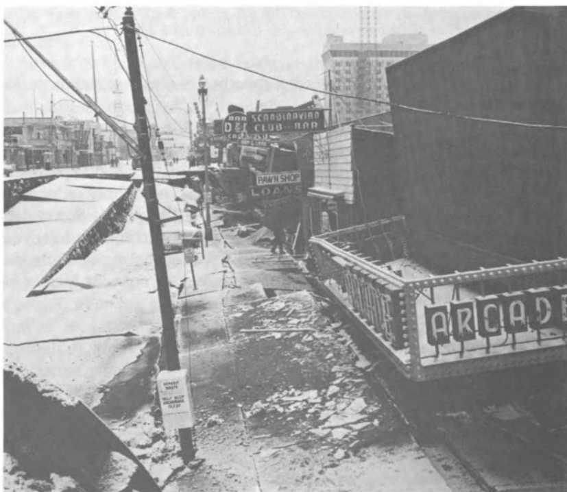
A large landslide during the 1964 Alaska earthquake caused extensive damage to these commercial buildings on Fourth Avenue. Research has done much to clarify the mechanism of such slides, but more needs to be done on assessing the potential for slides.
