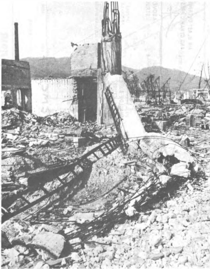
FIGURE 1 (5.34b) A circular, 60 feet high, reinforced-concrete stack at 0.34 mile from ground zero at Hiroshima (from The Effects of Nuclear Weapons , 1977).
