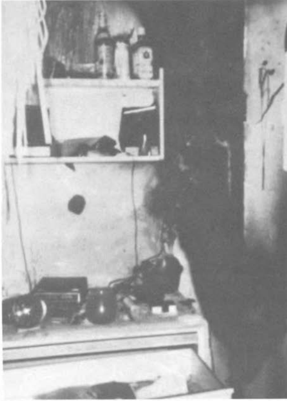
Figure 7.1.3. Representative shipboard fire damage.
