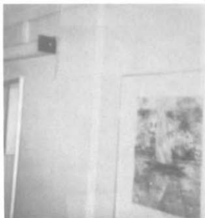
Figure 7.1.15. Undamaged stateroom beside hydraulic control room.
