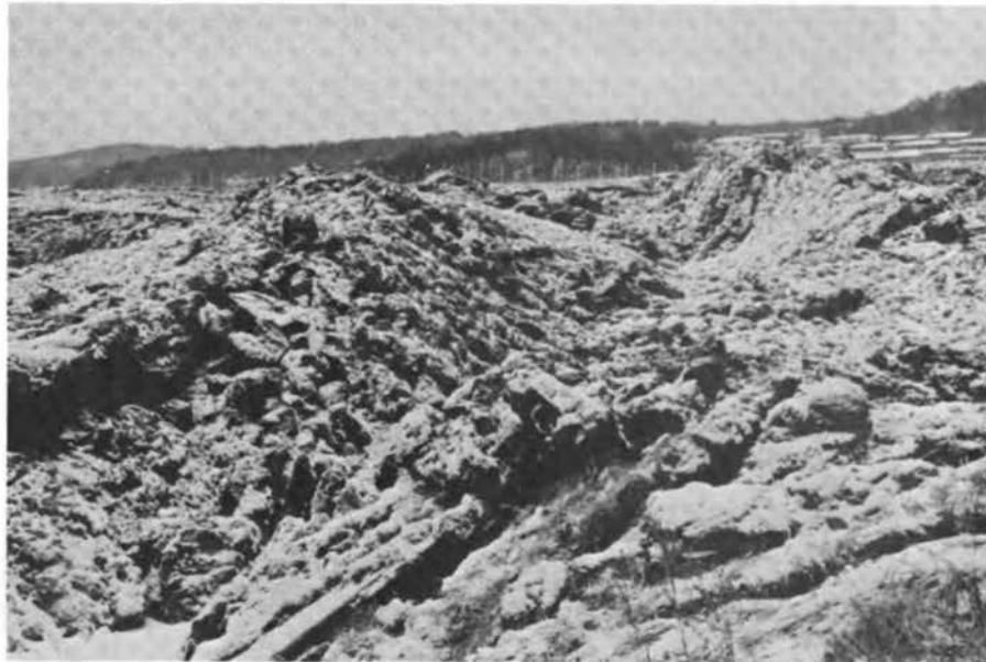
Fig. 9 Displacement of the road and heave and compression of the ground surface in the lower part of the slide.
