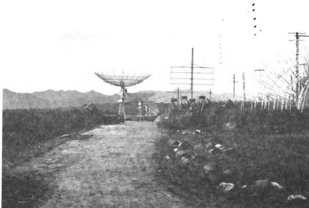
FIGURE 6 Radio antenna array at Mi-yun Station.
