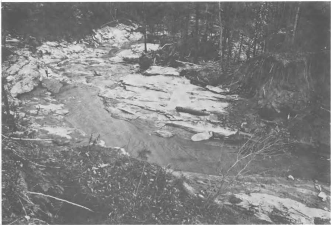
FIGURE 4b Scoured creek immediately downstream from dam looking downstream
