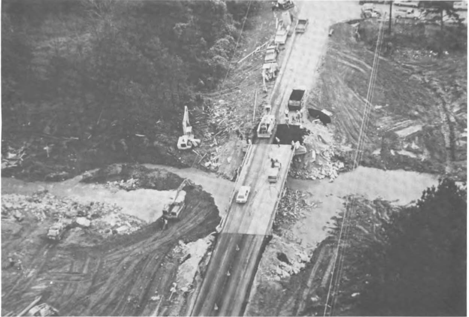
FIGURE 13 Highway 17 with new asphalt paving on new approach fills
