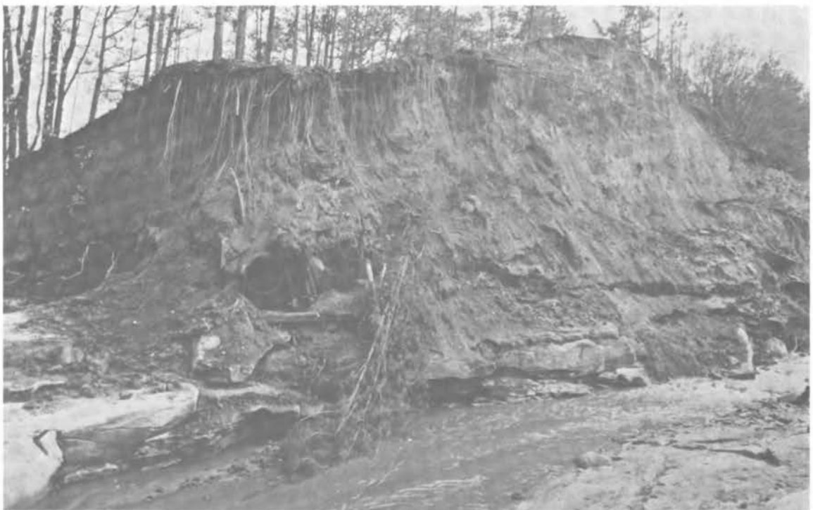
FIGURE 6 Face of breach on right side looking southwest, showing old penstock and remains of 1899 crib dam at downstream toe on left
