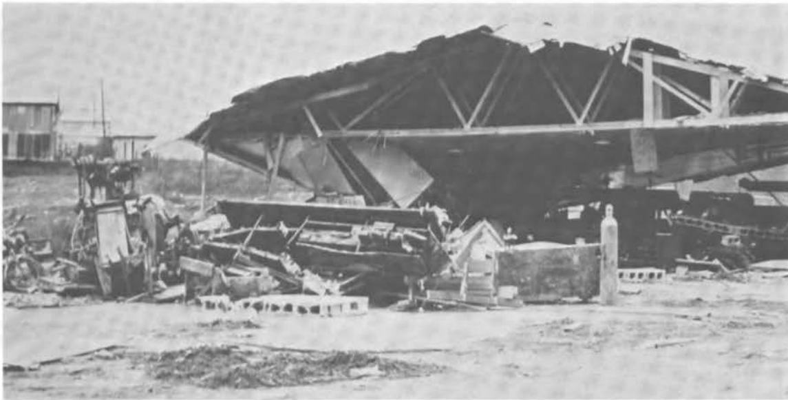
FIGURE 10a Maintenance garage and shop 1/2 mile downstream from dormitory looking downstream; creek to left
