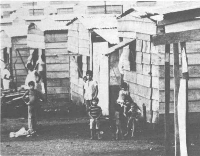
**FIGURE 9** *Low-Technology Solutions*: A total of 11,000 of these U.S. AID wooden housing units were built in Managua, Nicaragua, within 3 months of the disaster there. They were described as temporary when built, but they have inevitably become permanent.
