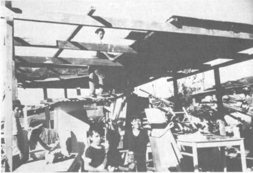
FIGURE 2 *Rapid Reconstruction*: This illustrates reconstruction in Zone 3 of Guatemala City 7 days after the earthquake.
