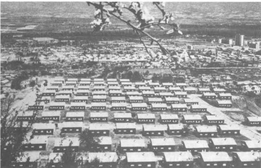
**FIGURE 10** *Prefabricated Housing*: These prefabricated housing units in Skopje, Yugoslavia, were built within 8 months following the earthquake of 1963.
