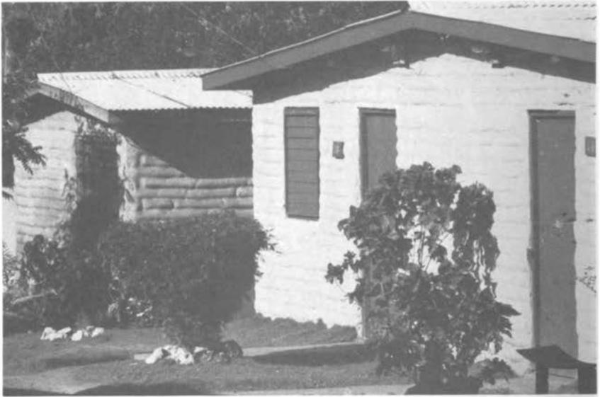
**FIGURE 7** *Self-Help Housing*: "Stack sack" housing is pictured in Masatepe, Nicaragua, 1974. This technique provides earthquake-proof construction, but the high cost of cement and burlap sacks limits its applicability by placing it out of range for poor families.
