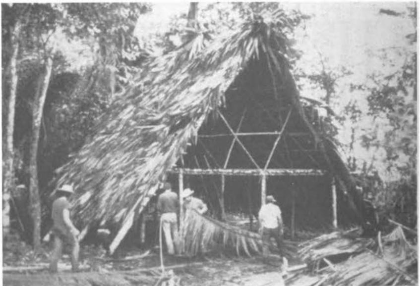
**FIGURE 8** *Low-Technology Shelter Solutions*: An example of low-technology solutions is the Intertect/Carnegie-Mellon University A-frame emergency housing shown here being field tested in Guatemala. The system was subsequently used in Bangladesh refugee camps.
