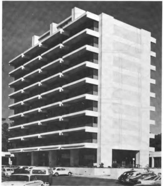
FIGURE 22 This Mississippi research building is a classic example of the simple horizontal overhang principle.
