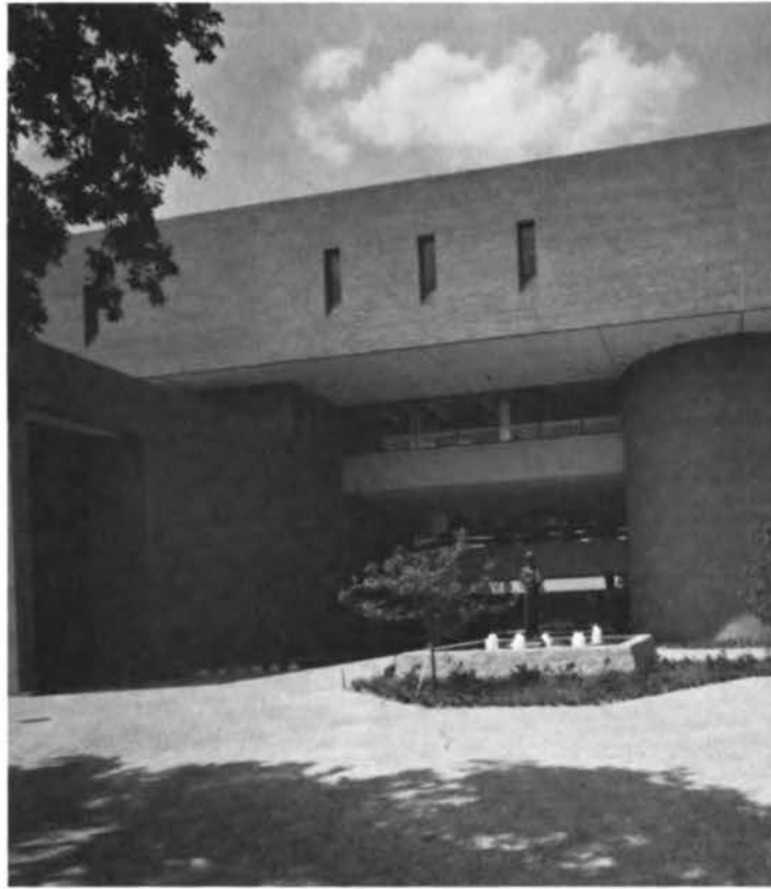
FIGURE 4 The Fine Arts Center of the University of Houston, Texas, has a breezeway entrance that provides a movement of air and ventilates the interior court.
