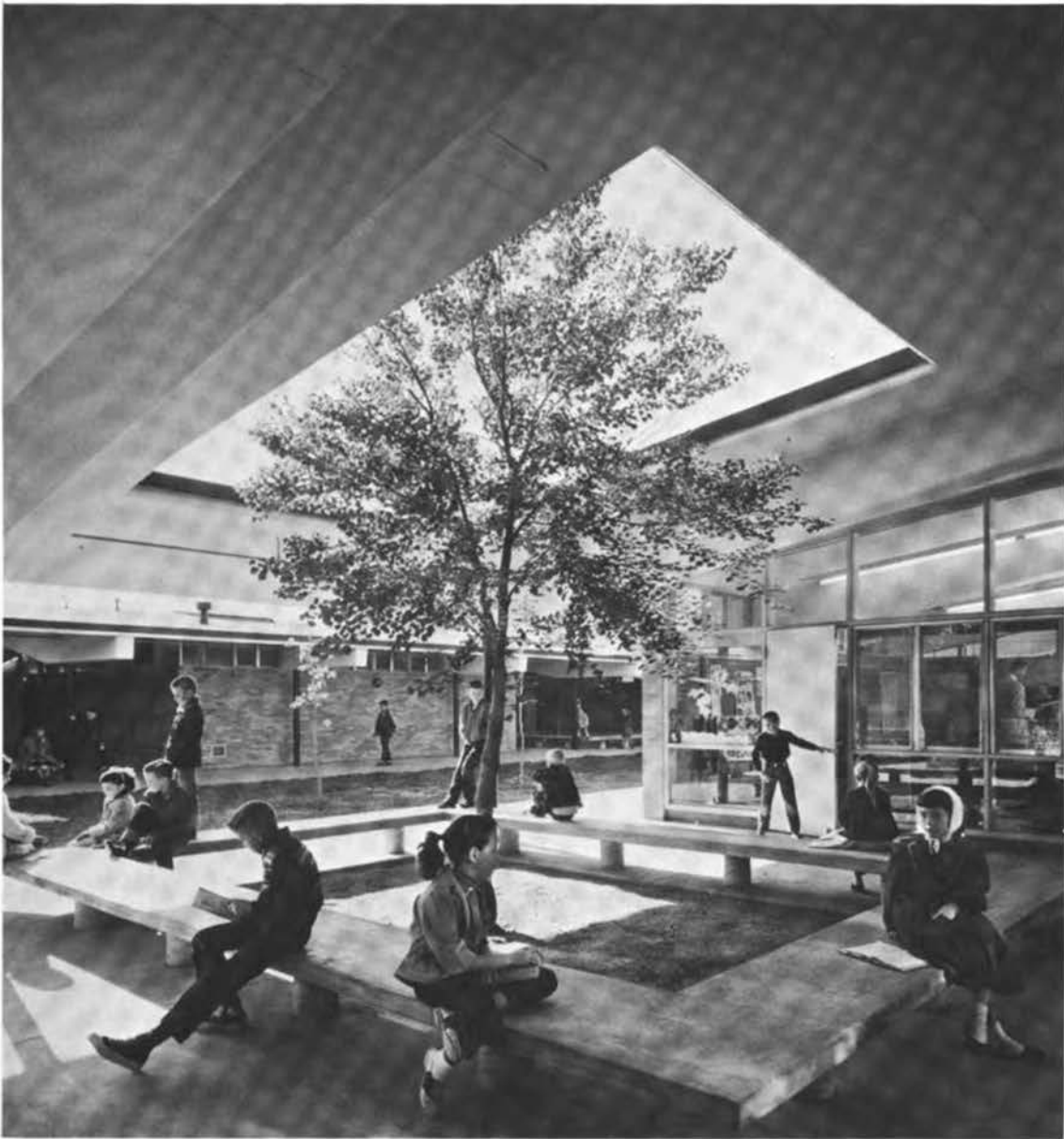
FIGURE 25 This partial roof provides needed sun protection for the students in this school while admitting enough daylight and direct solar radiation to maintain greenery.
