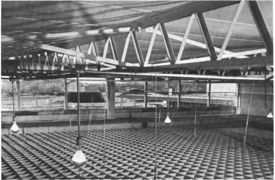
FIGURE 35 Classrooms in this school are lighted using a plenum that mixes and integrates natural and electric light.
