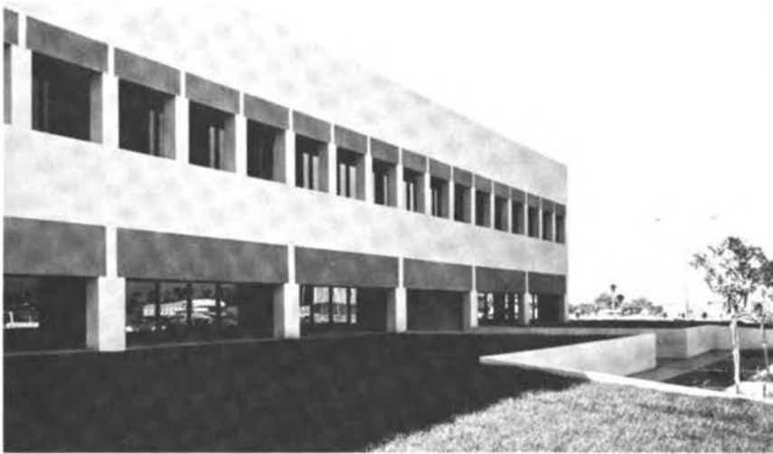
FIGURE 29 This technical school in Phoenix, Arizona, illustrates the application of earth berms to reduce heat loss by conduction.
