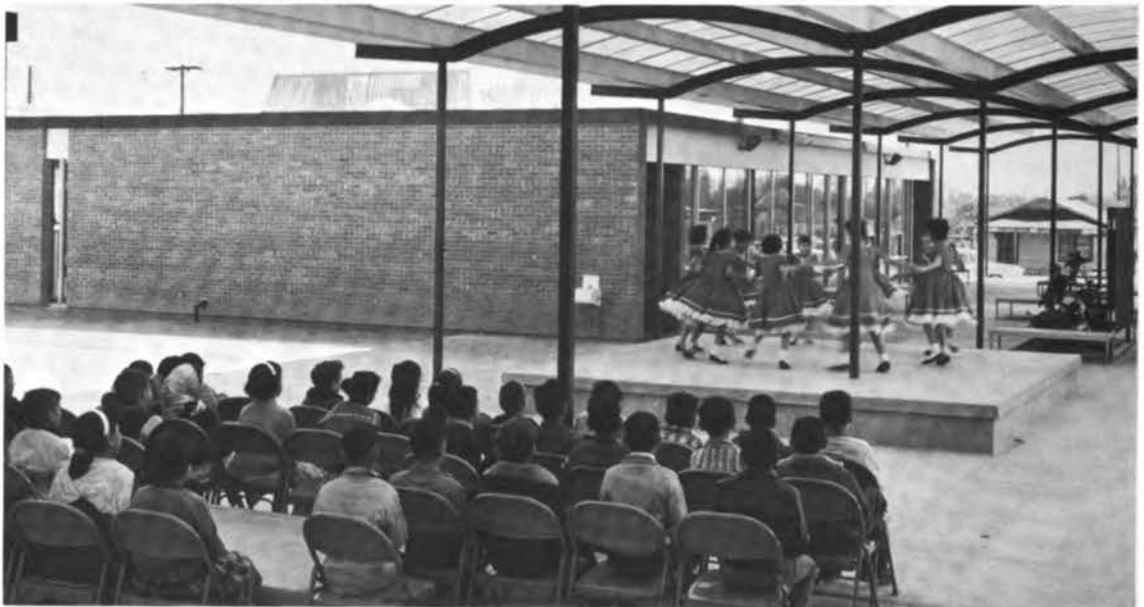
FIGURE 24 Sunlight is too intense for prolonged outdoor activities in Laredo, Texas, on the Mexican border, but this permanent roof blocks the direct sunlight while permitting natural daylight to filter through.
