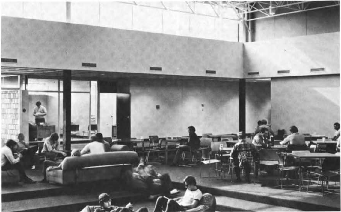
FIGURE 33 The clerestory arrangement in the student lounge at the Ohio Institute of Technology, in Columbus, provides the necessary natural light.
