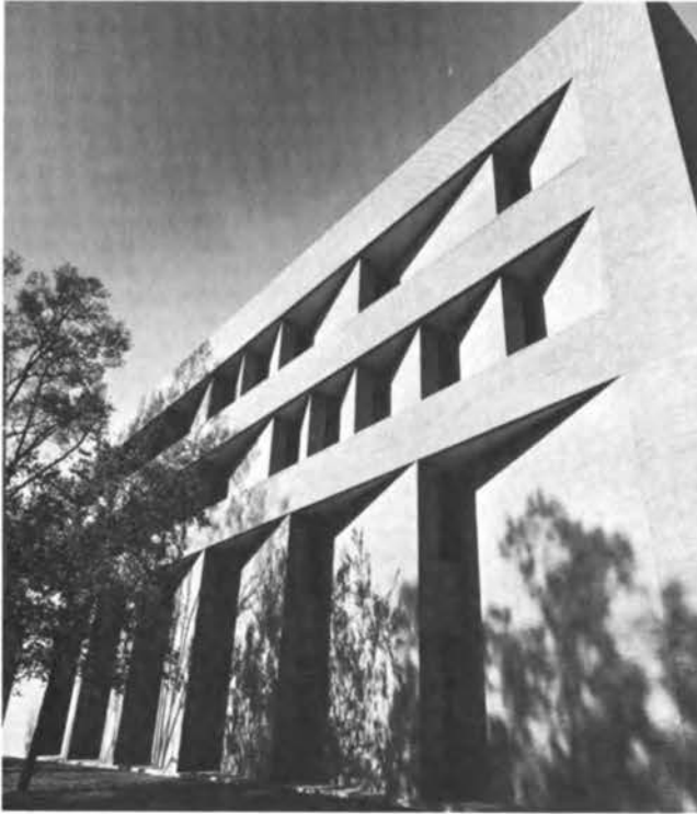
FIGURE 21 Fine Arts Center, University of Houston, Texas. Direct sunlight is totally eliminated from this building's interior, yet the sawtooth effect does permit natural daylight to enter.
