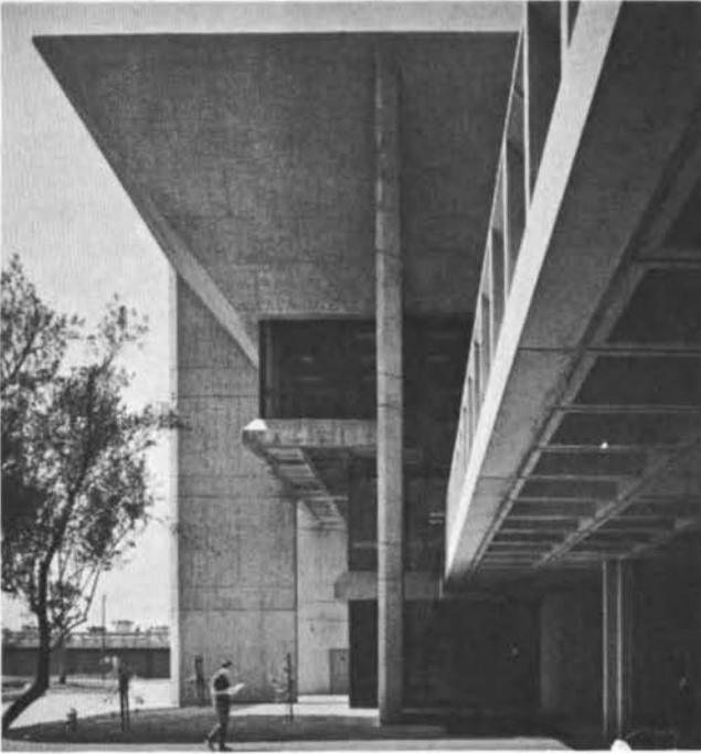
FIGURE 2 This building at a college in Southern California is a good example of the stepback method used to control the sun. The upper floors serve as overhangs to shade the lower floors. The soffit must be well insulated to ensure against heat transfer.
