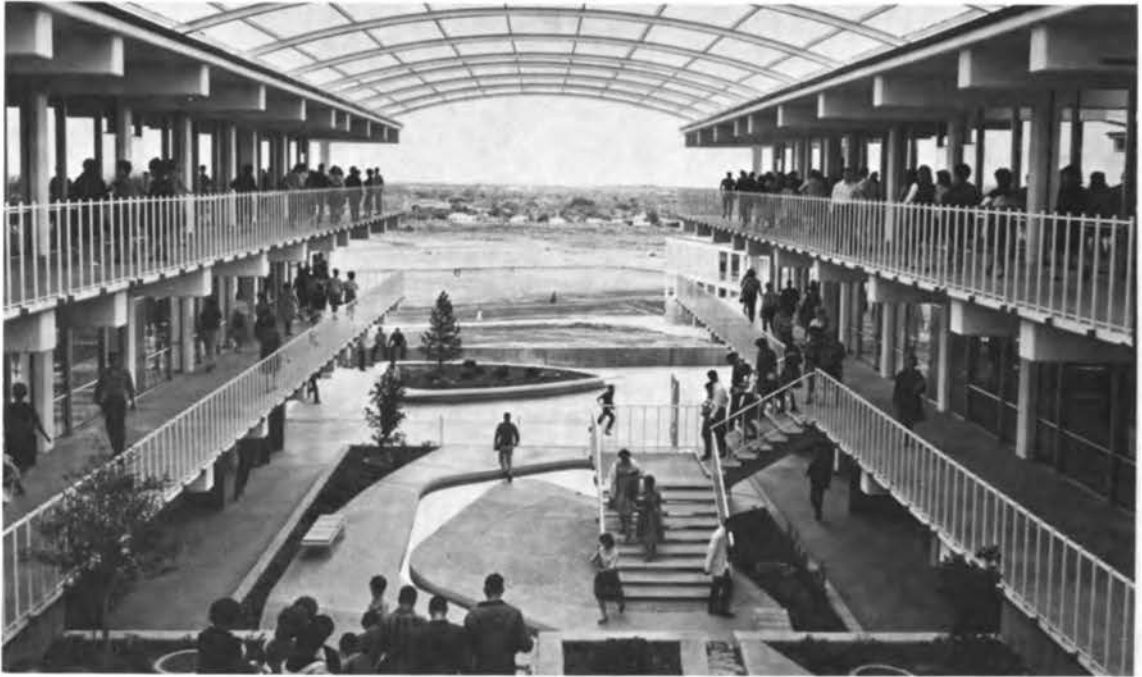
FIGURE 23 The umbrella type roof on the Carlsbad High School, in Carlsbad, New Mexico, permits the use of exterior corridors while protecting the students from direct solar radiation.
