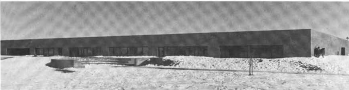
FIGURE 30 Insulation and scale were the primary reasons for using earth berms in the Mission Viejo Elementary School, Aurora, Colorado.
