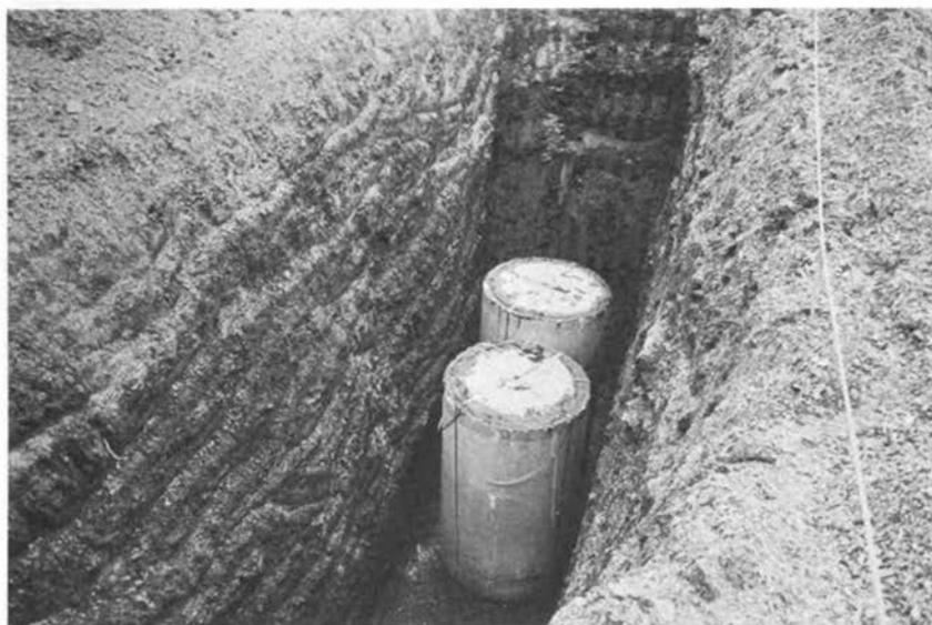
**FIGURE 11** Transuranium-contaminated waste at the Oak Ridge National Laboratory that has high gamma radiation levels is sealed in reinforced concrete casks 1.4 meters (4.6 feet) in diameter and 2.4 meters (7.9 feet) long having wall thicknesses from 12 to 30 centimeters (4.7 to 12 inches), depending on the shielding required. Casks are retrievably stored below grade in trenches 3 meters (10 feet) deep.
