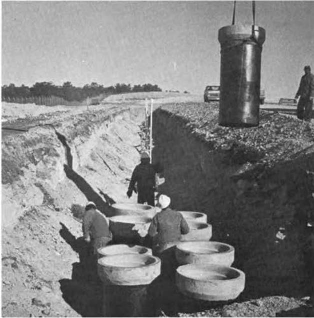
**FIGURE 16** Waterproofed concrete cylinders are placed into trenches ( $122 \times 9.2 \times 6.1$  meters, or  $400 \times 30 \times 20$  feet) in Area G at the Los Alamos Scientific Laboratory to retrievably store waste contaminated with plutonium-238. Topsoil is about 0.6 meters (2 feet) thick over tuff. The water table is 275 meters (900 feet) below the surface.
