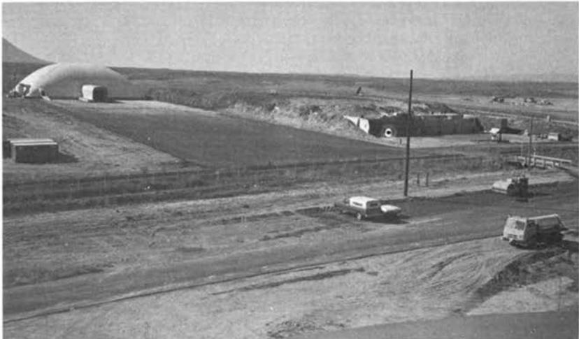
**FIGURE 8** On the left is shown an air support structure erected over the first cell of the second pad in the Transuranic Storage Area (TSA) at the Idaho National Engineering Laboratory. To the right is shown the final cell of the first pad being completed. Note that an airlock permits truck access to the air support structure without disturbing operations.
