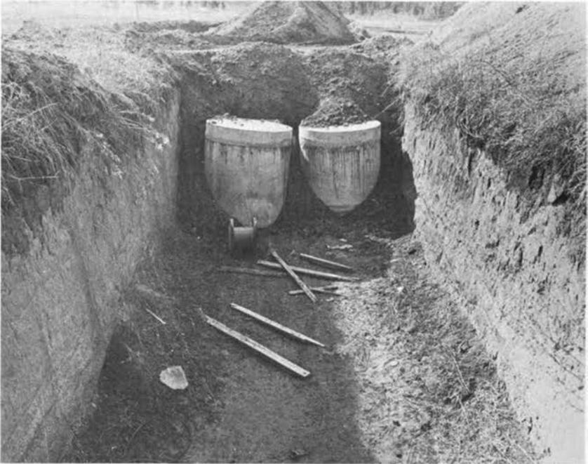
**FIGURE 14** Transuranium-contaminated waste in steel drums was originally sealed in concrete casks  $2 \times 2$  meters ( $6.6 \times 6.6$  feet) and retrievably stored in trenches up to 6 meters (20 feet) deep at the Savannah River Plant.
