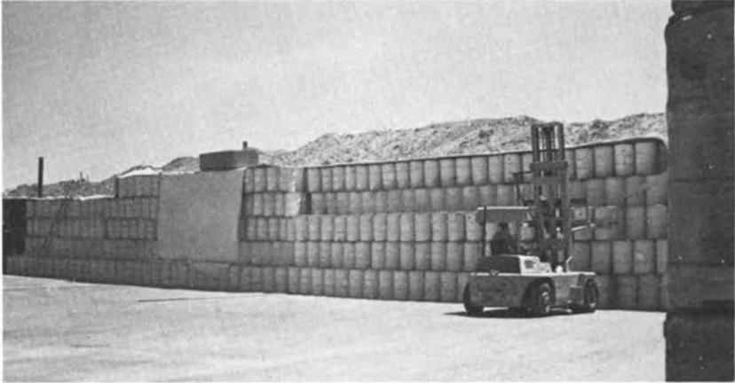
**FIGURE 7** Drums (210 liters or 55 gallons) of transuranium-contaminated waste are stacked on an asphalt pad at the Idaho National Engineering Laboratory in the Transuranic Storage Area (TSA) for retrievable storage. The drums and coated boxes are covered with flame-resistant plywood and reinforced plastic sheets before being covered by 1 meter (3 feet) of soil for protection from the weather.
