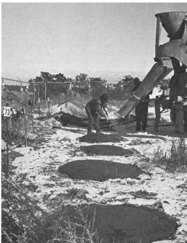
FIGURE 4 Shafts, 0.75 X 0.75 meters (2.5 X 2.5 feet), are drilled into the tuff in Area G at the Los Alamos Scientific Laboratory to dispose of solid waste that requires shielding. Some of the shafts are concrete lined. A sealing plug of concrete 1 meter (3.3 feet) thick is poured when the shaft is full.
