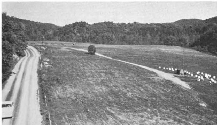
FIGURE 3 The Solid Waste Storage Area 4 at the Oak Ridge National Laboratory after it was no longer in use for burials. The burial area has been contoured and planted with grass. It occupies about 9.3 hectares (23 acres).
