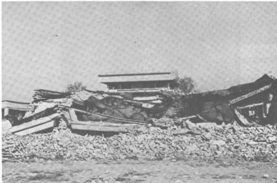
FIGURE 3.23 Northern End of the Main Clinic Building.
