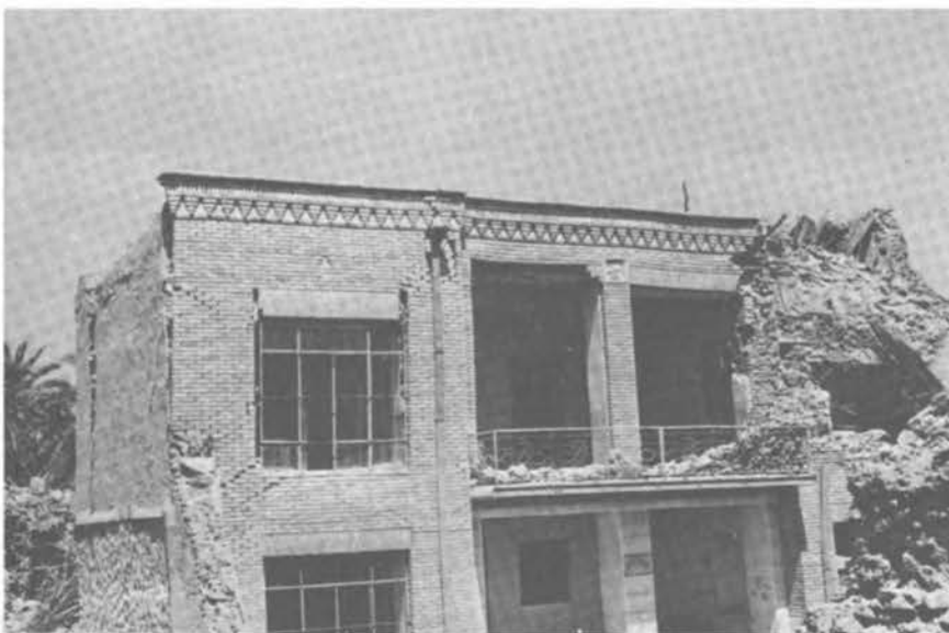
FIGURE 3.64 A Brick-masonry Building in the Village of Deh-beh.
