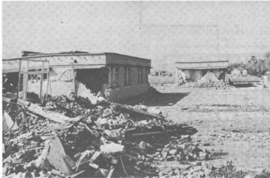
FIGURE 3.20 General View of the Qir Clinic After the Earthquake.
