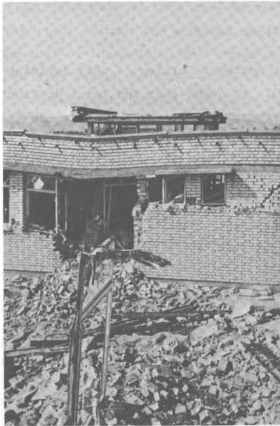
FIGURE 3.22 Western End of the Main Clinic Building.
