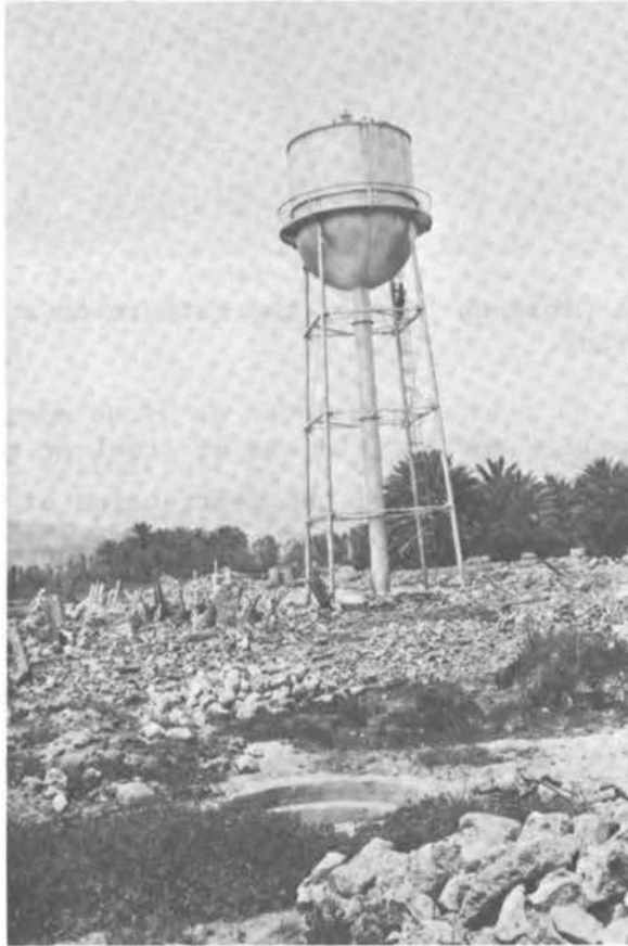
FIGURE 3.32 Q̄ir Water Tank After the Earthquake.
