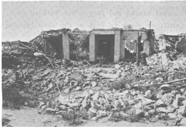
FIGURE 3.65 Flexural and Shear Cracks at the End of Lintels and Columns (Village of Deh-beh).
