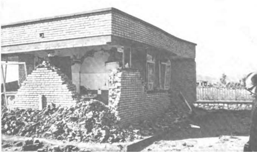
FIGURE 3.26 The Southwest Corner of the Garage-Janitor Building.
