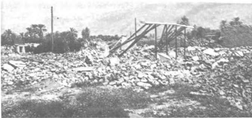
FIGURE 3.60 The Ruins of Another Building in Qir Where a Portion of the Roof was Supported by Steel Columns.
