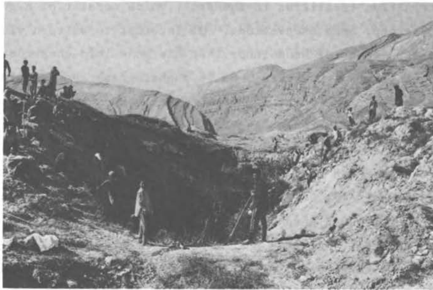
FIGURE 3.87 A Team of Laborers Cleaning Out One of the Slumped-in Open Excavations.
