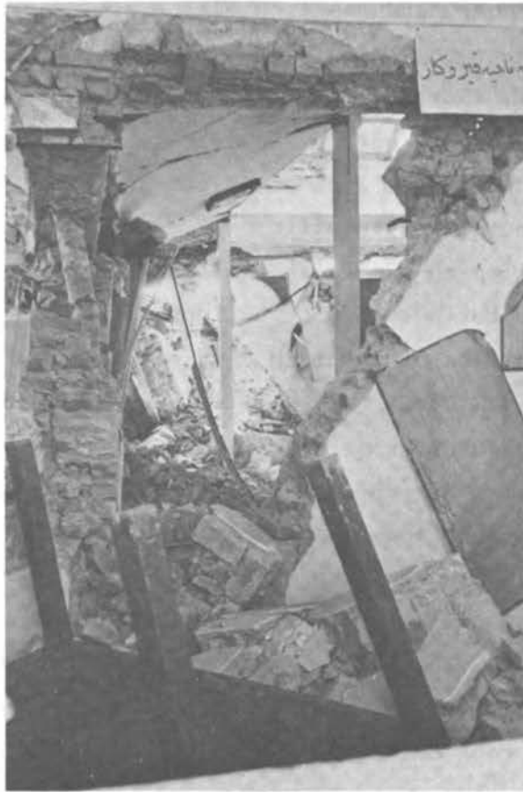
FIGURE 3.25 A View of the Interior Steel Columns Supporting the Roof of the Main Waiting Hall and the Adjacent Roofs.
