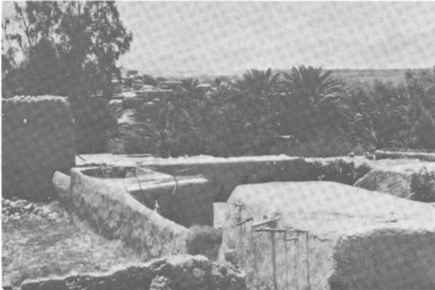
FIGURE 3.13 Some Typical Adobe Houses in the Village of Lāghar.
