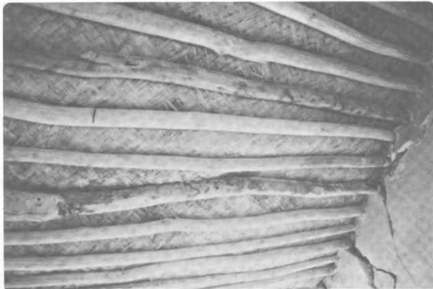
FIGURE 3.16 Inside View of a Typical Flat Timbered Roof in Qīr.
