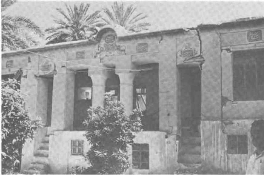
FIGURE 3.67 A Brick-masonry House in the Village of Deh-beh.
