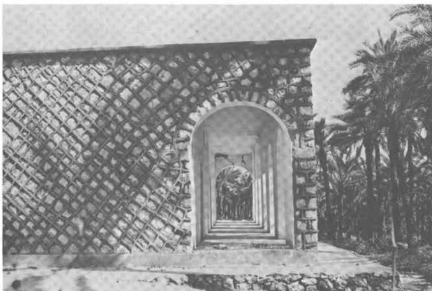
FIGURE 3.47 West-end View of the Ābe Garm School.
