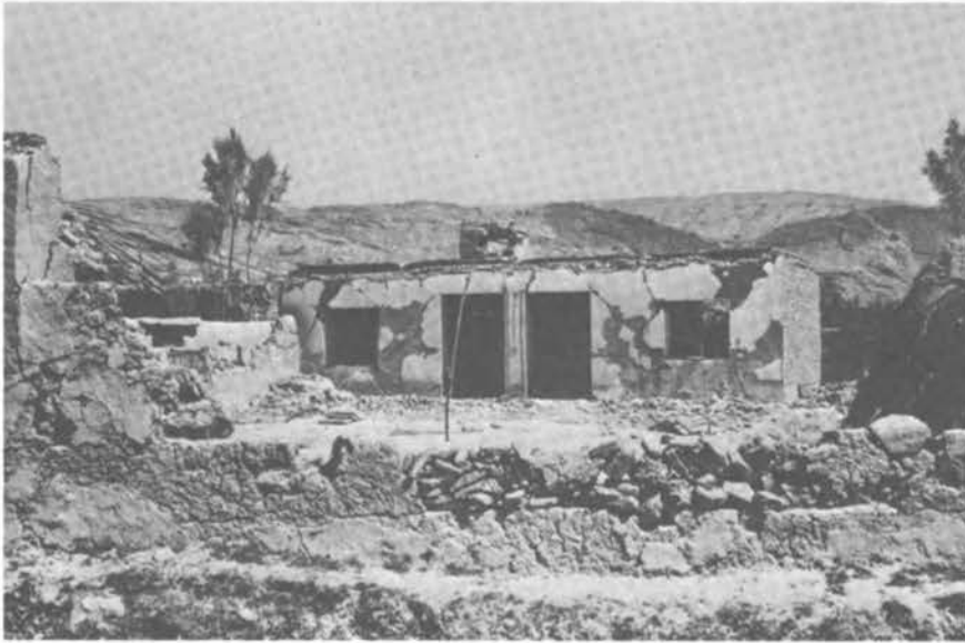
FIGURE 3.63 Typical X-shaped Shear Cracks and Flexural Cracks on the Walls of a Symmetrical Adobe Building.
