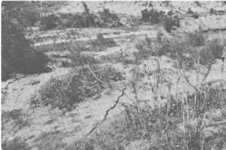
FIGURE 3.84 Typical Cracking and Slumping of the Banks of the River Qara-Aqaj Near the Shāhābad Bridge.
