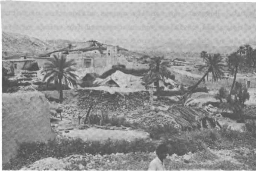
FIGURE 3.73 Typical In-Plane Failure of the Exterior Walls of a Stone-Masonry Building in the Village of Kamasej.
