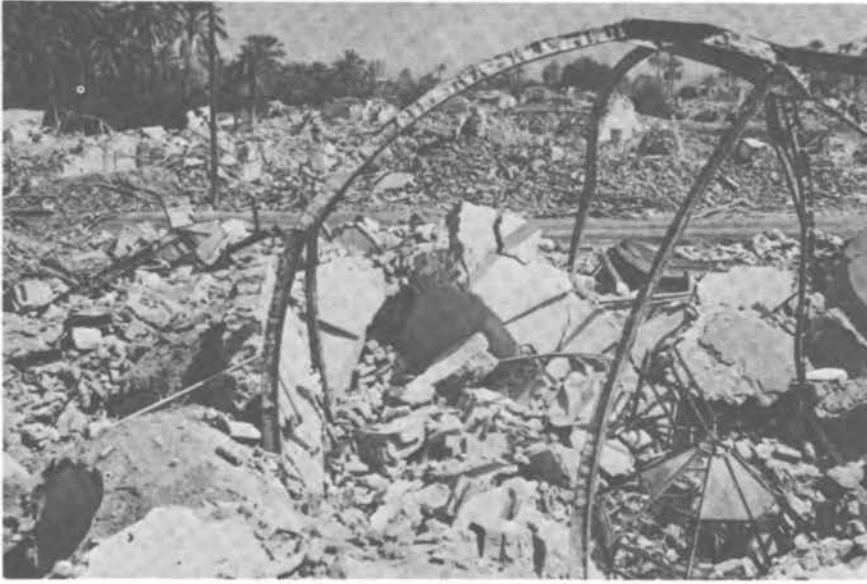
FIGURE 3.56 A Close-up View of the Destroyed Dome of the Qir Bathing House.
