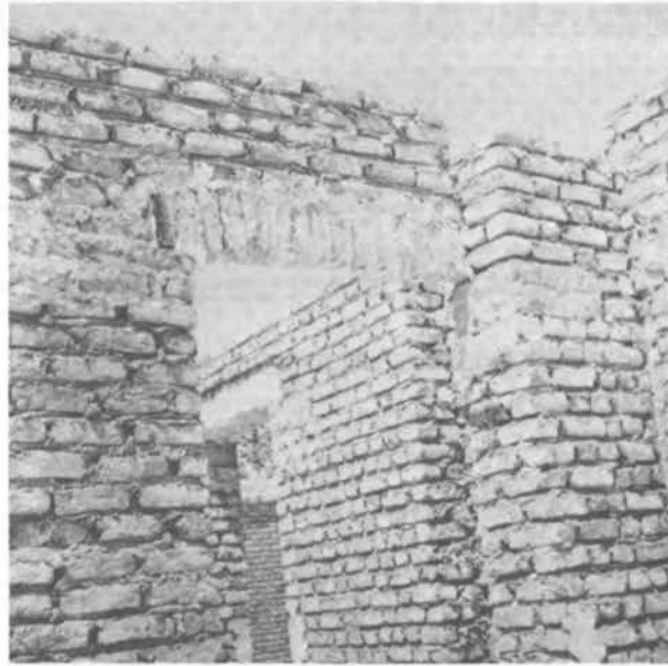
FIGURE 5.2 A Typical Brick-Masonry Wall of a Residential Building in Shiraz.
