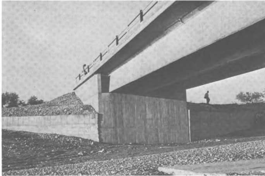
FIGURE 3.36 The Western Abutment of the Bridge and the Retaining Walls.
