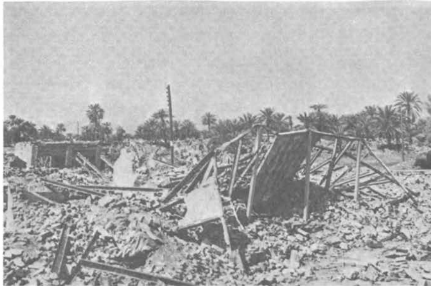
FIGURE 3.59 The Ruins of a Building in Qir Where Part of its Roof was Supported by Steel Columns.
