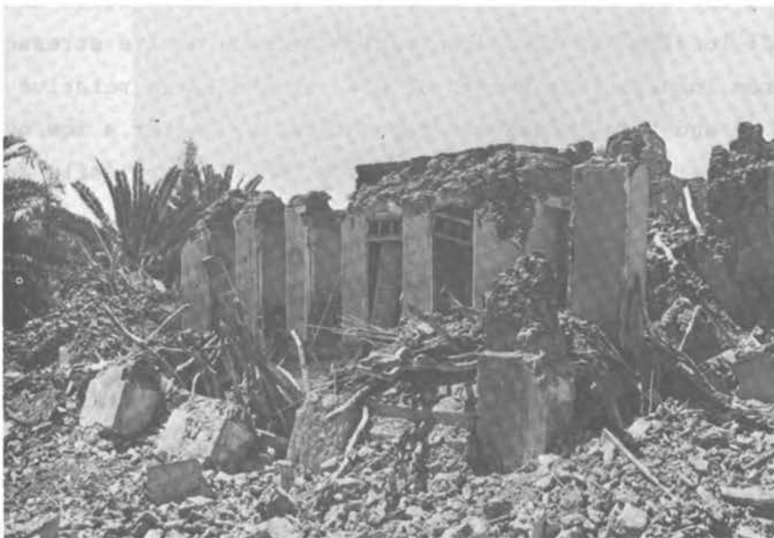
FIGURE 3.72 Typical Failure of the Arched or Timbered Lintels with Insufficient Bearing Length on the Supporting Walls.
