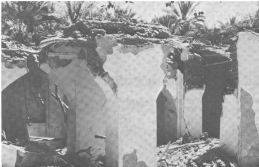
FIGURE 3.66 Typical Shear Failure of the Arched Lintels of a Mosque in Qir.
