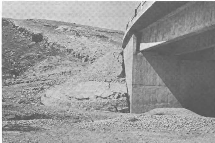
FIGURE 3.37 The Eastern Abutment of the Bridge and the Retaining Walls.
