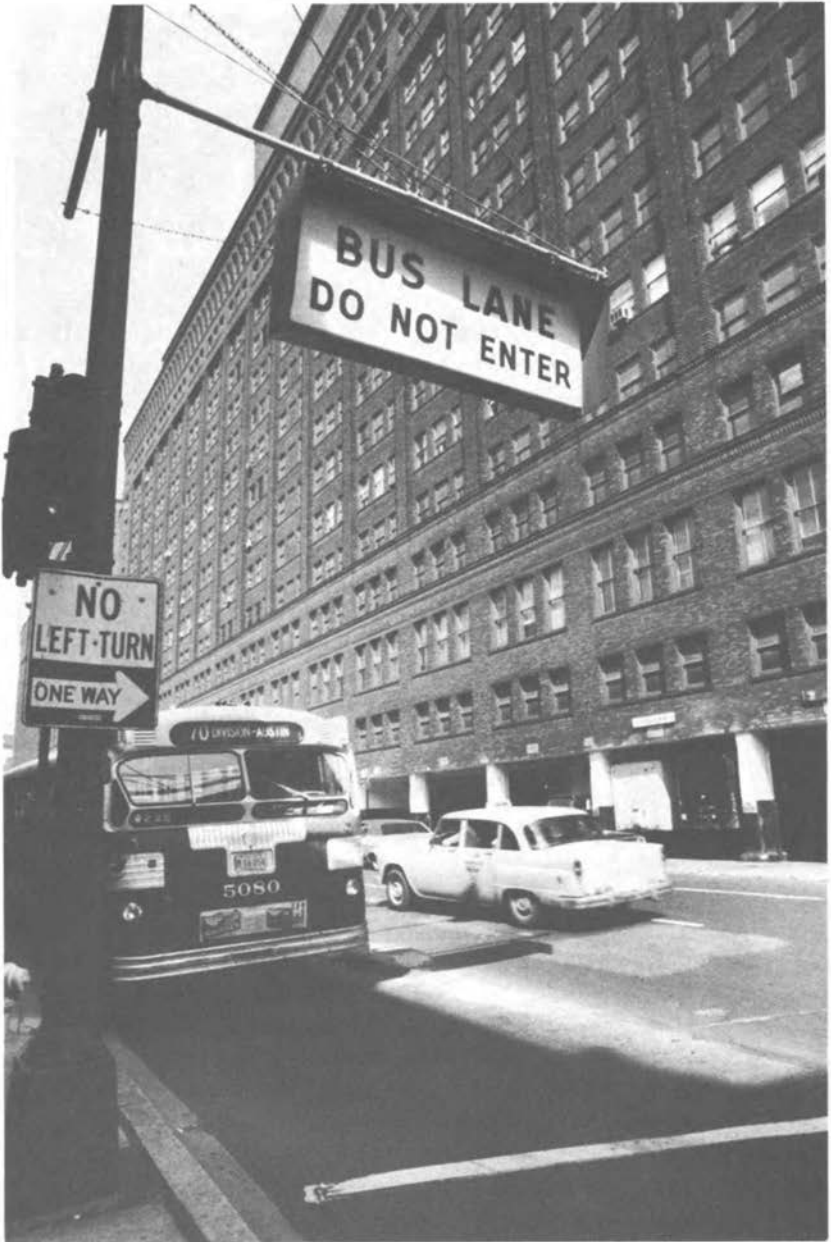
FIGURE 10 Exclusive reverse bus lane permitting passengers to exit at train loading platform.
