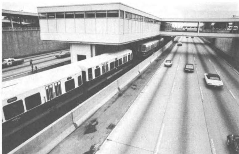
FIGURE 4 Terminal located within median strip, the Dan Ryan 95th Street Station.
