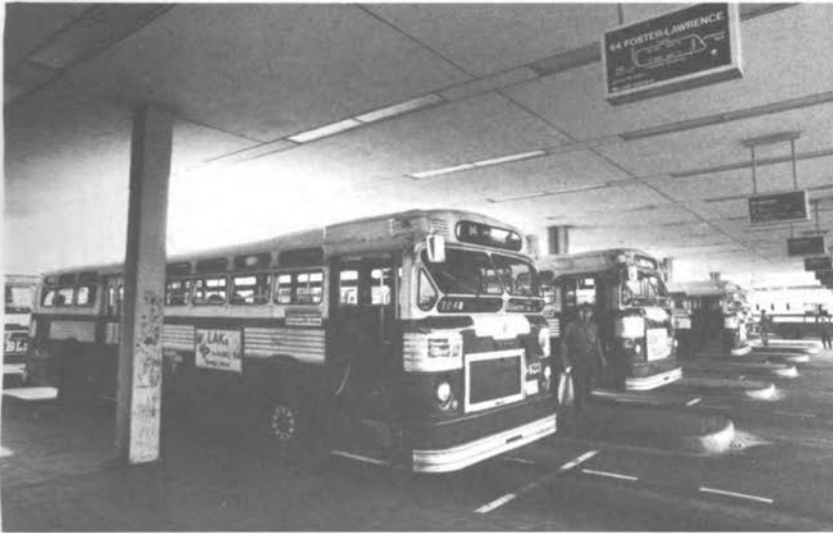
FIGURE 5 Common loading bay, Jefferson Park Terminal, Kennedy Expressway.
