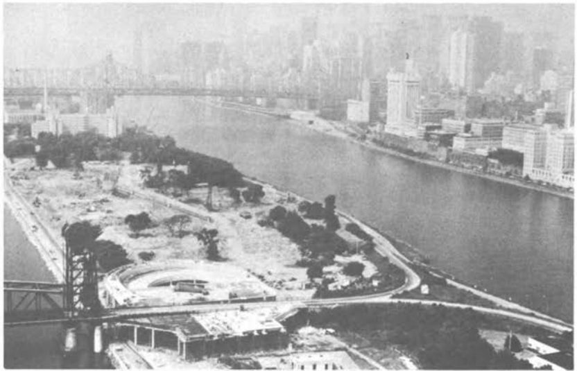
FIGURE 17 Parking terminal ramps under construction.
