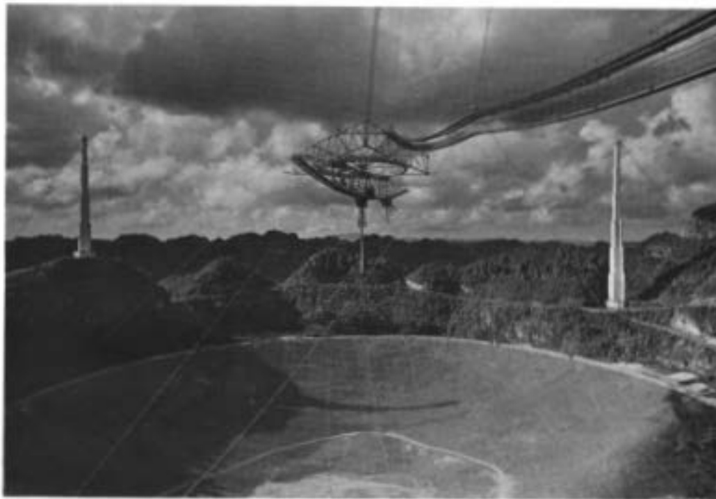
The 1000-ft radio telescope at Arecibo, Puerto Rico, is capable of communicating with a similar instrument at a distance of 1000 light-years. (Photo courtesy of National Astronomy and Ionosphere Center.)
